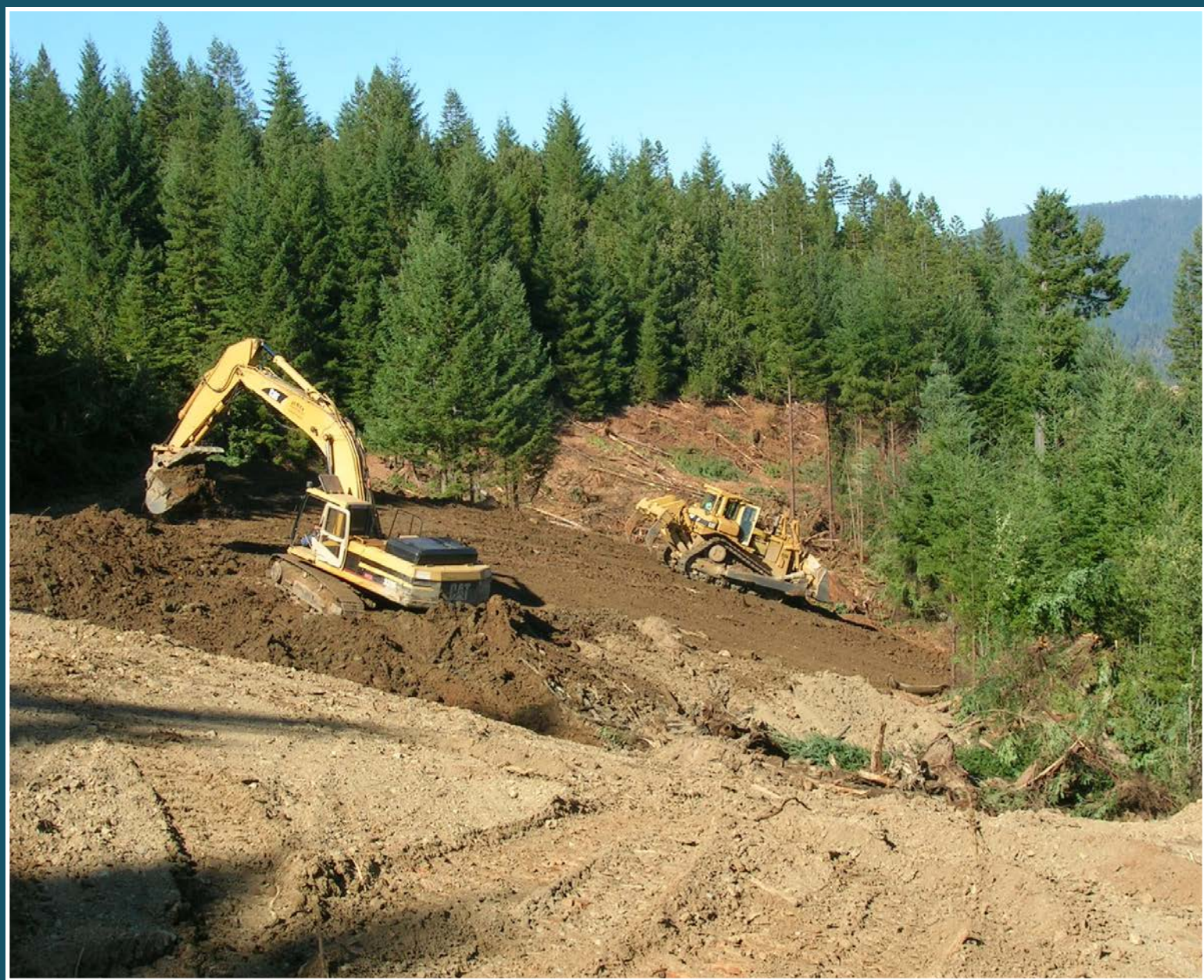
Excavation team at work. An excavator and bulldozer work together on a stretch of road to recontour natural hillslope topography and drainage patterns.
