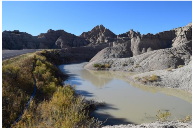
Figure 4. Ponding caused by clogged culvert to north side of road on Dillon Pass section at MP 25
