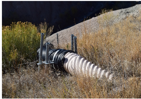
Figure 7. Example of temporary down drain and metal pipe to be removed and replaced
