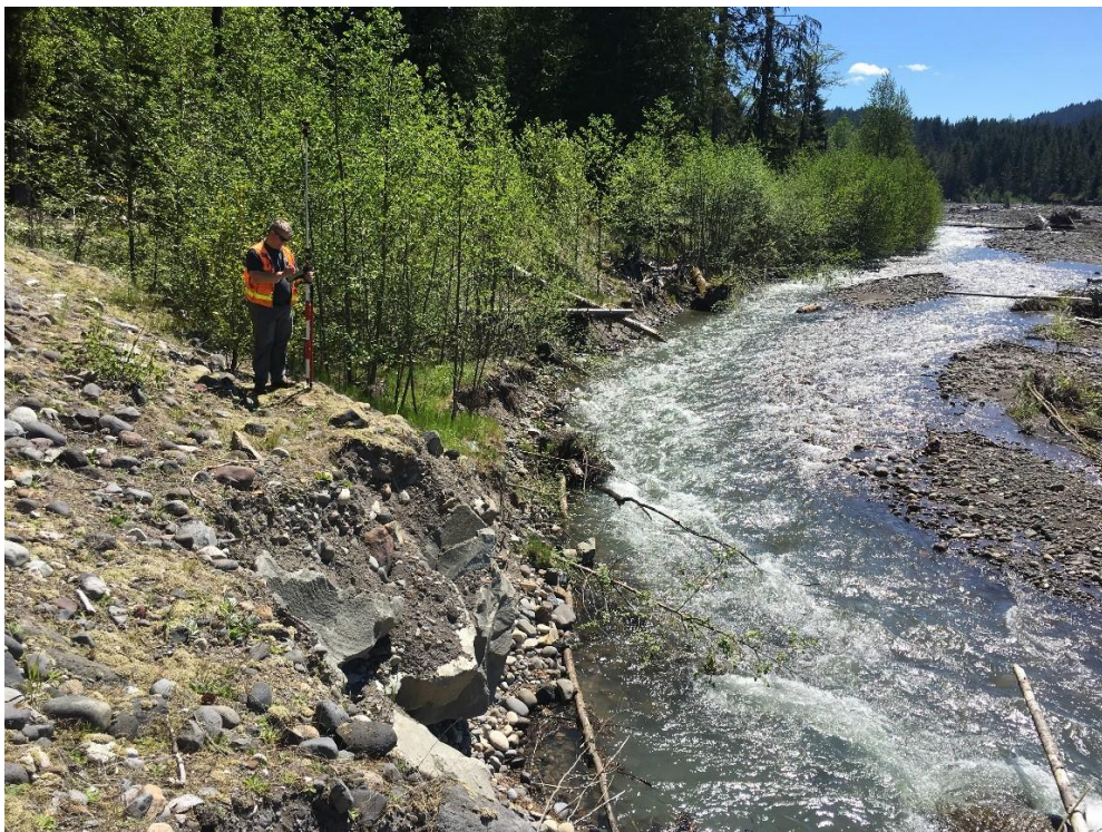
Upstream end of project, closer look at damaged toe and face scour
