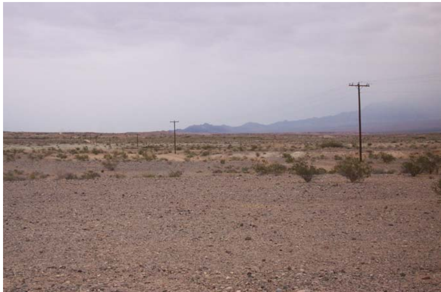
Figure 4. Existing power line with horizontal pole top configuration.
