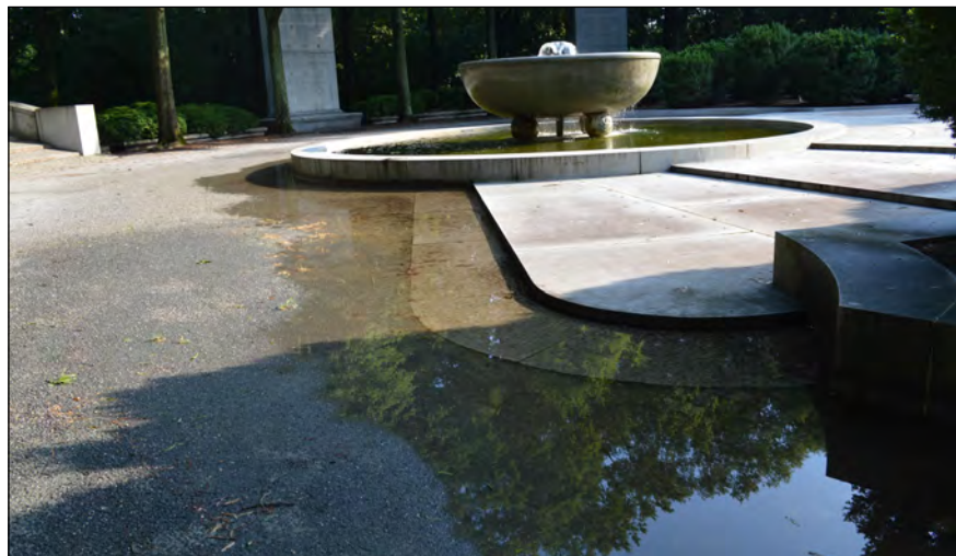
Figure 165. Resulting pooling from clogged drains, 2016. (JMT)
