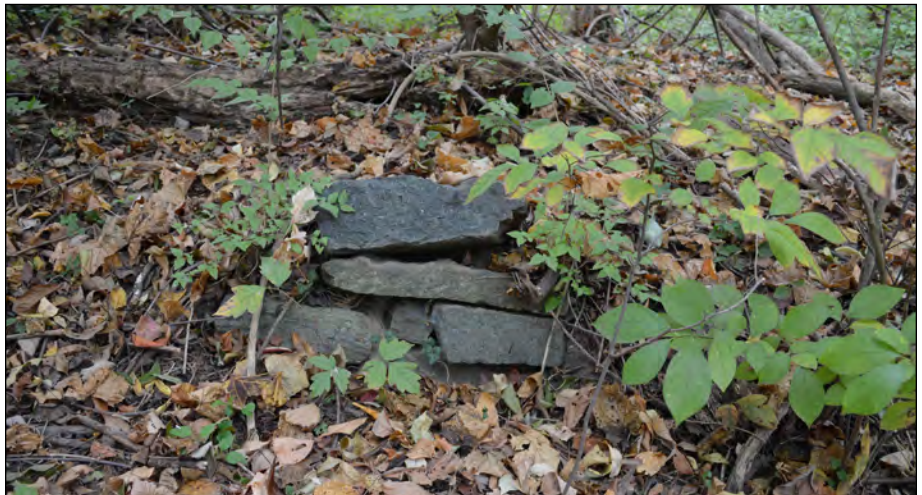
Figure 107. Dry laid stone retaining wall on the south end of the island, 2016. (JMT)
