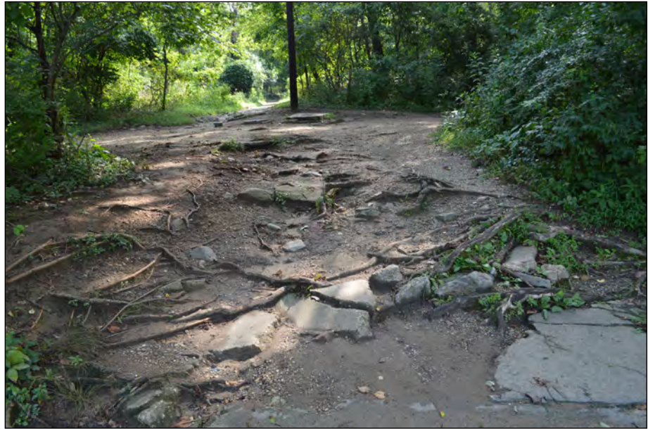
Figure 62. Concrete and stone causeway remnants. Severe erosion caused by tree root growth and people walking visible, 2016. (JMT)
