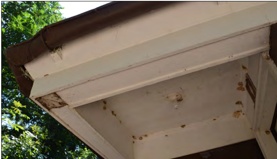
Figure 99. Missing roof support pier at entrance to women's room of comfort station, 2016. (JMT)
