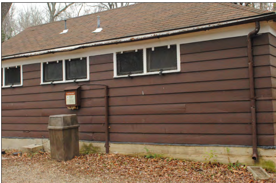
Figure 100. Damage to gutters, downspouts, and siding of comfort station, 2016. (JMT)
