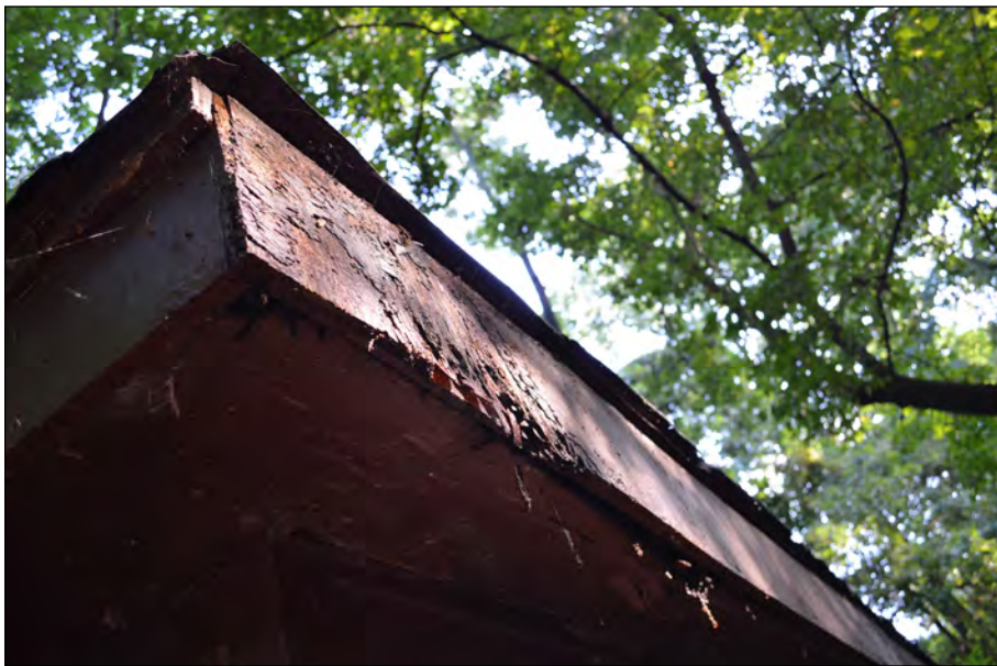
Figure 104. Storage building roof fascia board showing peeling paint and wood rot, 2016. (JMT)
