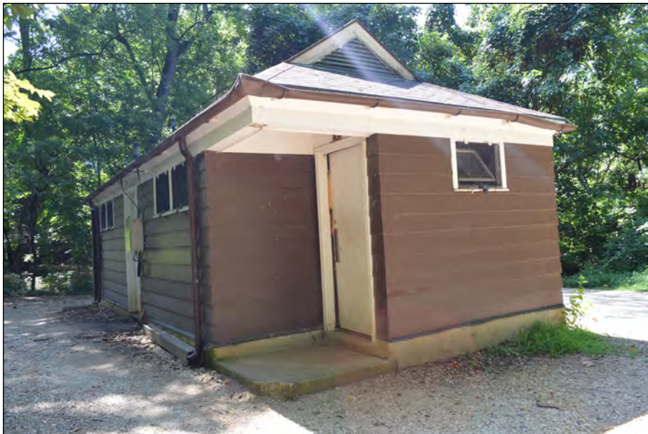
Figure 94. Northeast corner of comfort station showing access to women's room; note the missing roof support pier, 2016. (JMT)
