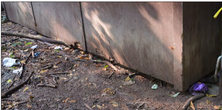
Figure 105. Water damage at the base of the storage building, 2016. (JMT)
