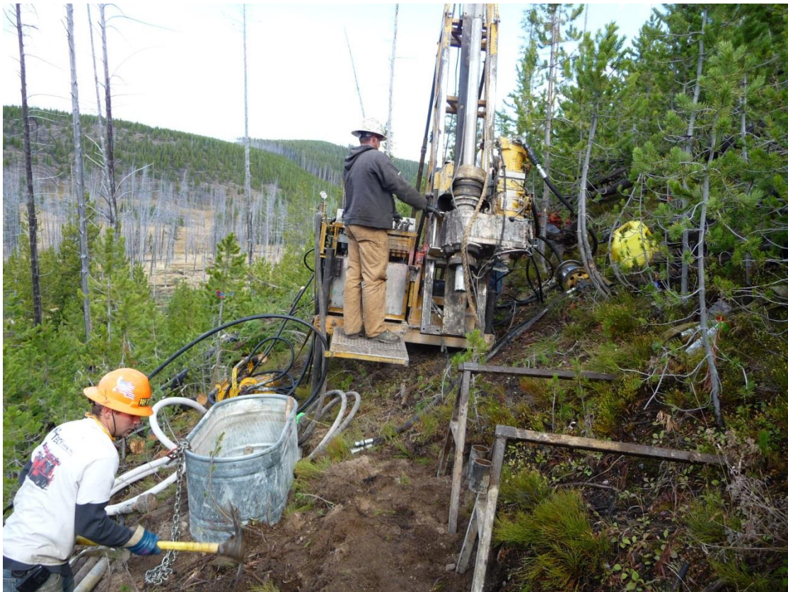
Figure 4. Typical helicopter or crane portable geotechnical drilling operation.
