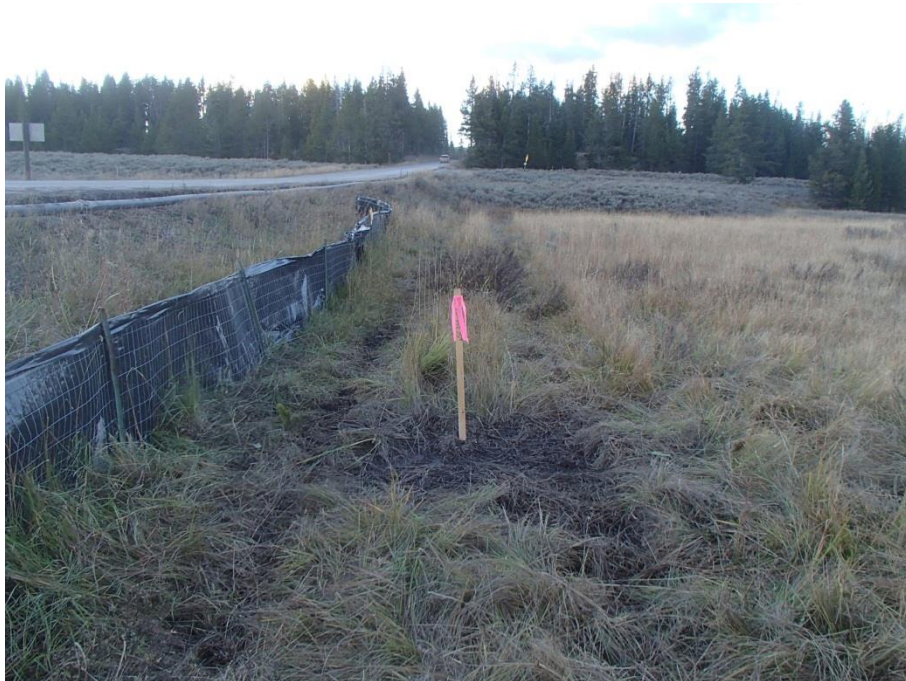
Figure 3. An example of wetland impacts following a track-mounted drilling operation in a wetland environment.
