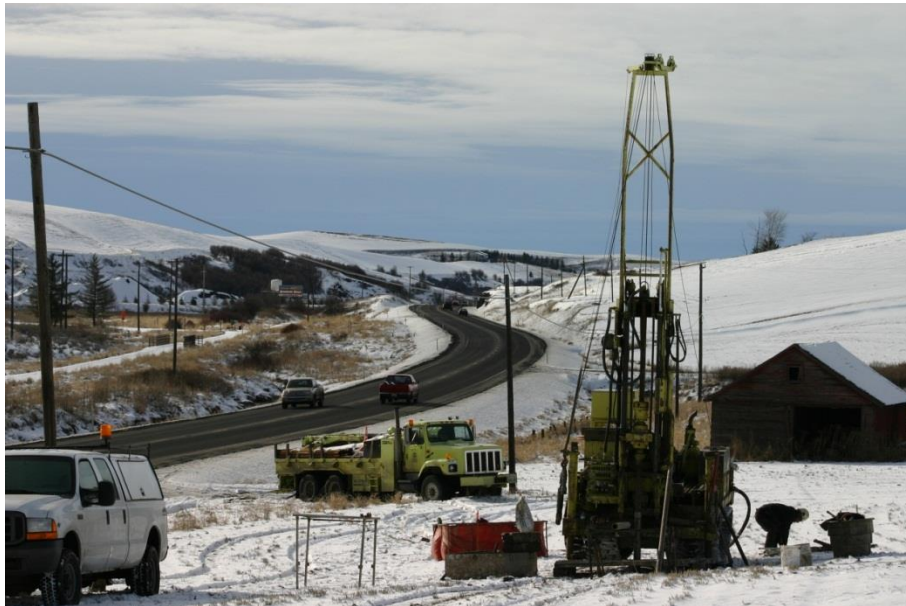
Figure 2. Typical track-mounted geotechnical drilling operation.
