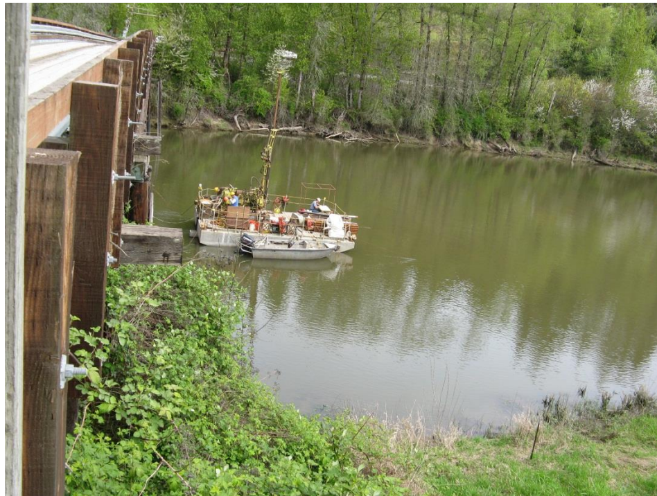
Figure 5. Typical pontoon barge with skid-mounted geotechnical drilling operation.
