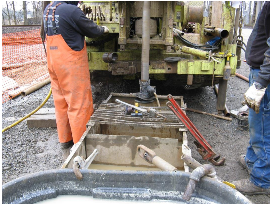
Figure 6. Use of a baffled tub to contain returning drill fluids laden with sediment during the drilling process.
