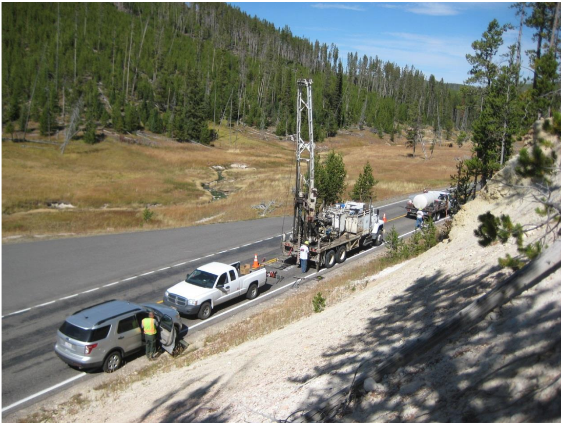
Figure 1. Typical truck-mounted geotechnical drilling operation
