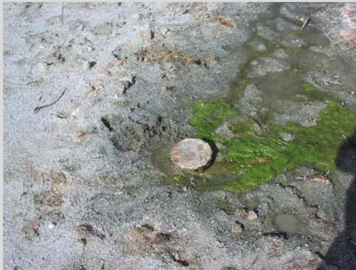
Watson Well is a capped drilled well
