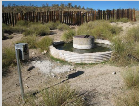
Cut Spring is piped from a springbox to a concrete drinker
