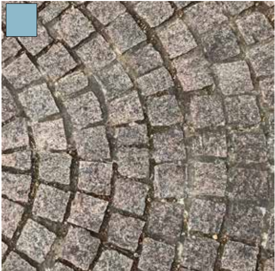
GRANITE SETTS: COLDSRING CARNELIAN GRANITE SETTS
