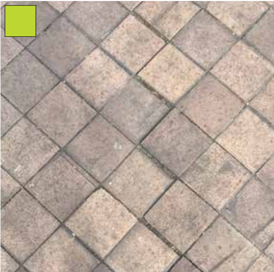
PENNSYLVANIA AVENUE PAVER: TERRA COTTA PAVERS AND BRICKS OF VARYING SIZES
