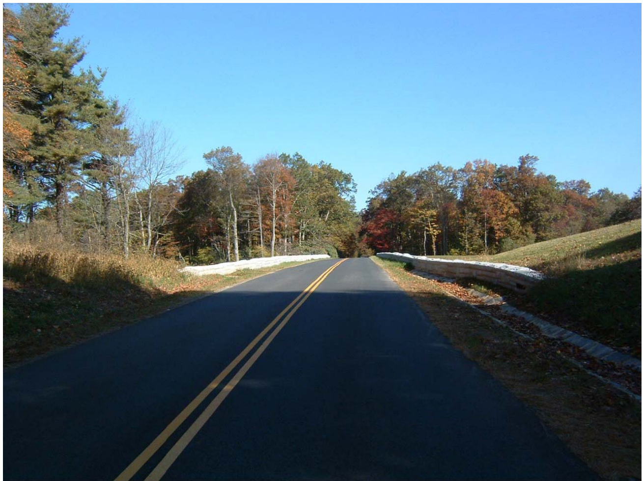
Figure 6. Alternative D: example of a bridge similar to proposed bridge. The proposed bridge would look most like this bridge along the roadway with class B masonry parapet walls and guardwall approaches. The bridge in the photo has grassed shoulders over the bridge span and along the guardwall approaches. The proposed bridge would have class B masonry parapet and guardwall approaches with grassy shoulders that would be continuous.
