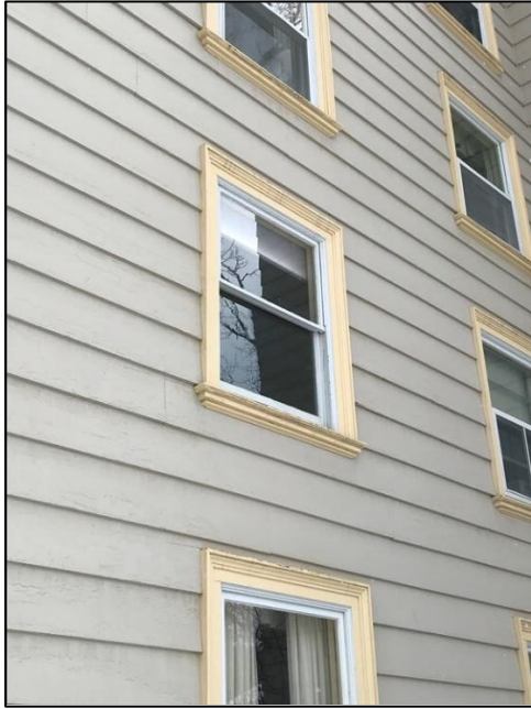
Figure 3: Exterior photos of existing one-over-one, double-hung, wood windows on the Mammoth Hot Springs Hotel Guest Wing (the bottom sash screen has been removed to get a better view of the window). Existing windows on the Guest Wing of the Mammoth Hot Springs Hotel have screens on the bottom sash only. The tops of the double hung windows are painted shut. Photos show the character of the painted trim.
