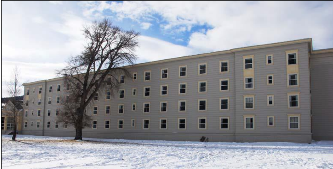
Figure 1: Existing view of east side of the Guest Wing of the Mammoth Hot Springs Hotel that is finished with wide horizontal shiplap siding. Window openings are uniformly spaced on each of the elevations. The windows are one-over-one, double-hung and are finished with projecting cornice with architrave trim. There are decorative panels between the head of the 3rd floor windows and the sill of the 4th floor windows.
