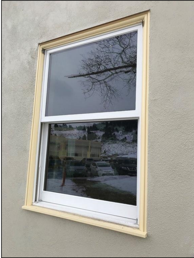
Figure 5: Exterior photos of a new one-over-one, double-hung, wood window that was used on a recent building addition to the 1937 two-story portion of the Mammoth Hot Springs Hotel that has a stucco exterior. Windows on this portion of the hotel have a different style of trim. The park proposes to use this type of window to replace the existing one-over-one, double-hung, wood windows on the Guest Wing, which has a horizontal lapped wood siding exterior. The trim on the new Guest Wing windows would match the exterior trim of existing Guest Wing windows as shown in Figure 1 through Figure 4. These new windows would have full height wood screens that cover both sashes so the upper sash can be lowered to achieve better ventilation in the guest rooms. Photo on the left is without a screen, photo on the right has a screen.
