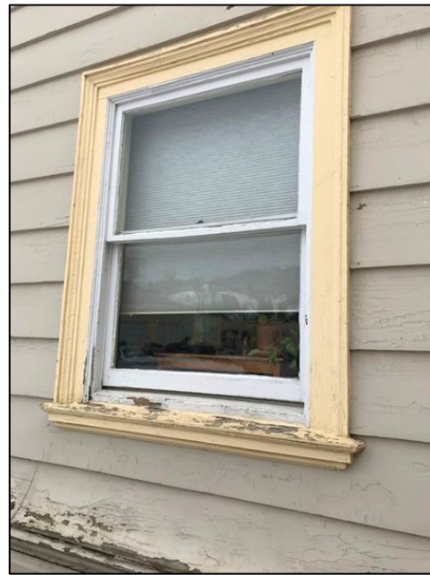
Figure 3: Exterior photos of existing one-over-one, double-hung, wood windows on the Mammoth Hot Springs Hotel Guest Wing (the bottom sash screen has been removed to get a better view of the window). Existing windows on the Guest Wing of the Mammoth Hot Springs Hotel have screens on the bottom sash only. The tops of the double hung windows are painted shut. Photos show the character of the painted trim.
