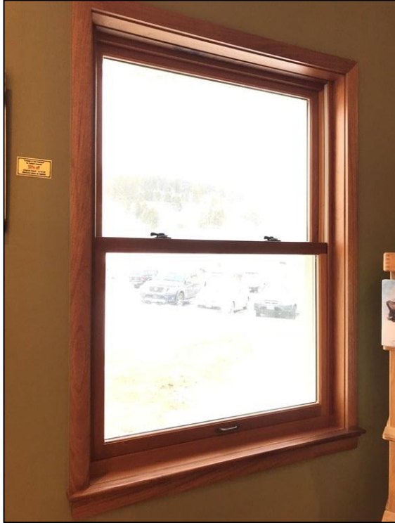
Figure 6: Interior photo of the new one-over-one, double-hung, wood window that was used on a recent building addition to the later, 1937 two-story portion of the Mammoth Hot Springs Hotel. Please note the interior trim on this window in this photo has a different style of trim and is unpainted. These new windows would be painted and use trim that matches the interior trim on the existing painted windows as shown in Figure 4 .
