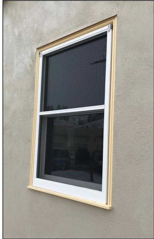
Figure 5: Exterior photos of a new one-over-one, double-hung, wood window that was used on a recent building addition to the 1937 two-story portion of the Mammoth Hot Springs Hotel that has a stucco exterior. Windows on this portion of the hotel have a different style of trim. The park proposes to use this type of window to replace the existing one-over-one, double-hung, wood windows on the Guest Wing, which has a horizontal lapped wood siding exterior. The trim on the new Guest Wing windows would match the exterior trim of existing Guest Wing windows as shown in Figure 1 through Figure 4. These new windows would have full height wood screens that cover both sashes so the upper sash can be lowered to achieve better ventilation in the guest rooms. Photo on the left is without a screen, photo on the right has a screen.
