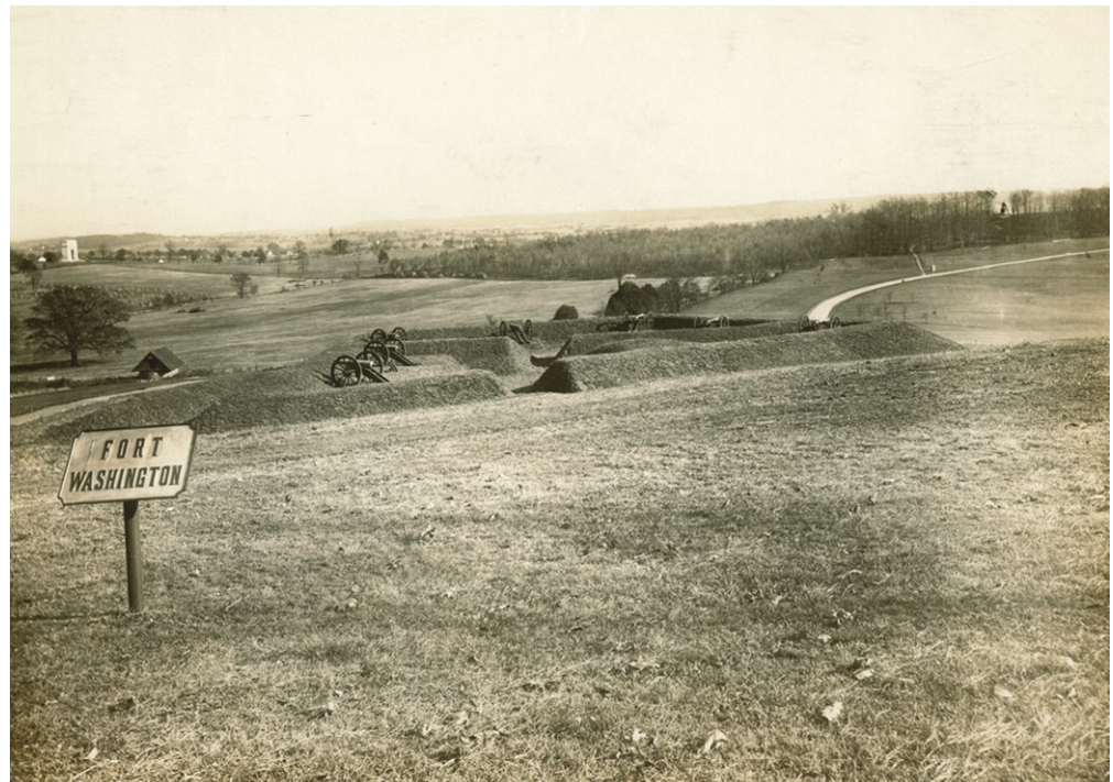
The Valley Forge Park Commission modified the existing agricultural landscape into a stylized commemorative landscape. Visible from left to right are the National Memorial Arch, the reconstructed Fort Washington, Outer Line Drive, and the General Wayne Statue in Wayne's Woods.
