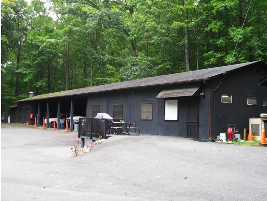
War Department Maintenance Building – Chief Ranger's Office New insulation, underlayment and 30-year architectural asphalt shingle roof and ridge vent will be installed
