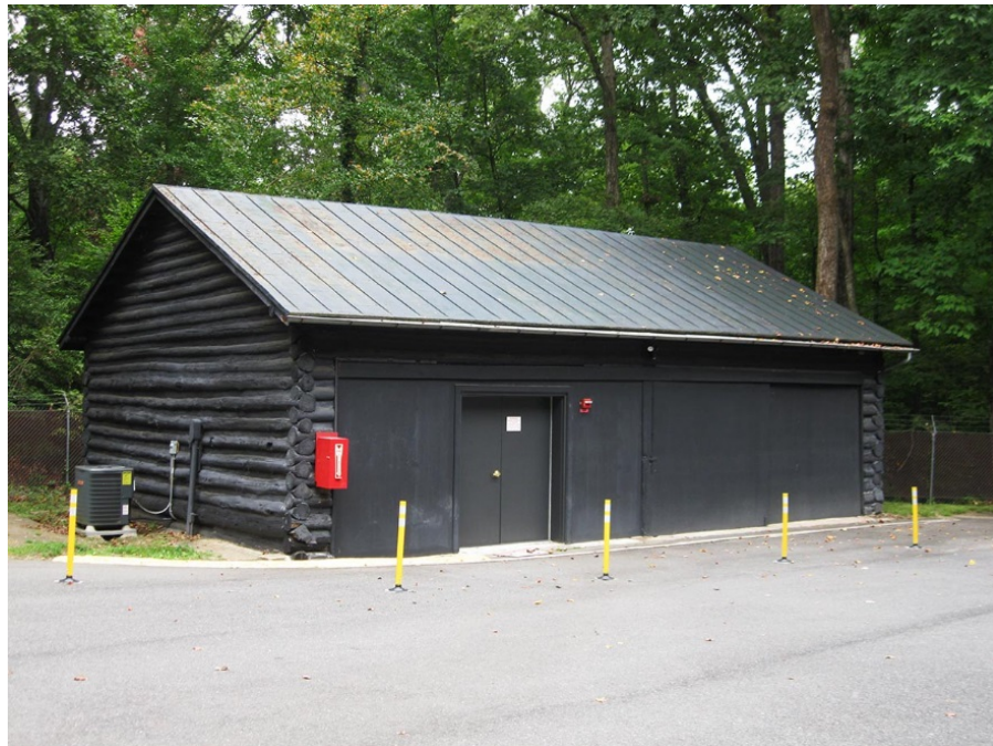
War Department Log Garage – Curatorial Storage Rehabbed by some scrapping of flaking paint and an overall new coat of paint.
