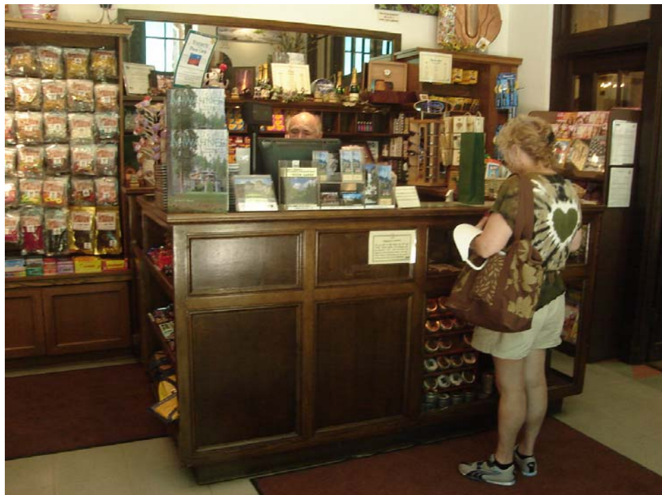
Photo 2 Ahwahnee Sweet Shop showing the current, non-ADA compliant counter
