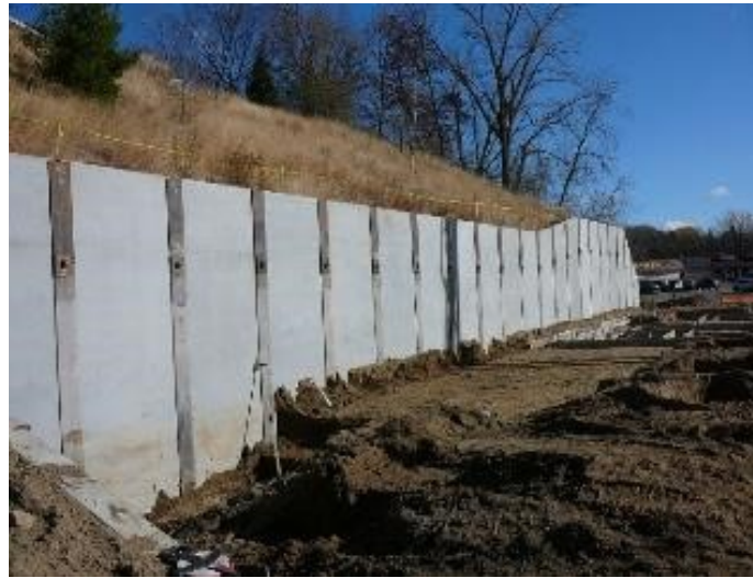
FIGURE 3. EXAMPLE SOLDIER PILE WALL
