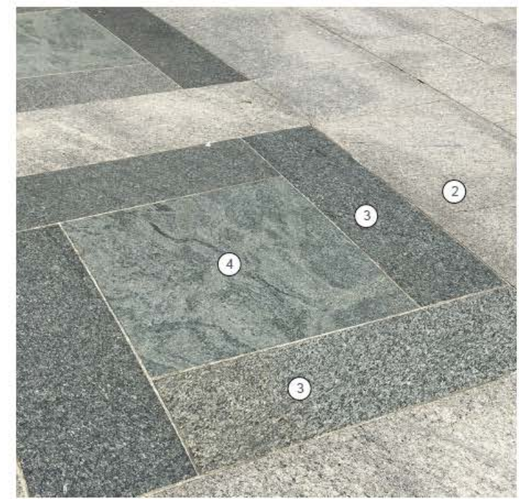
Paving pattern detail showing four types of stone used at WWII Memorial
