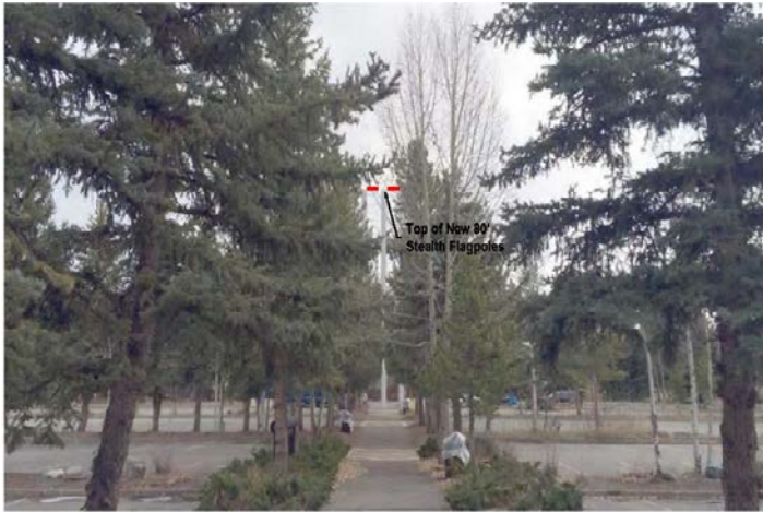
Photo Simulation of 80' Stealth Flagpole Towers with Interior Antennas and Equipment Shelter at Jackson Lake Lodge (view to the east from the lodge)
