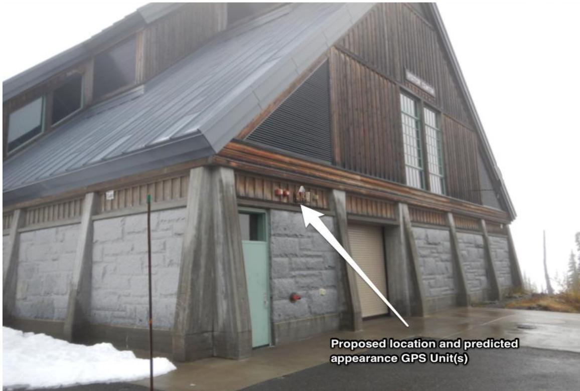
**Figure 11.** Proposed location of GPS unit(s) on the west end of the JVC. A shroud matching the exterior siding would mask the GPS units. One unit would be installed per carrier.
