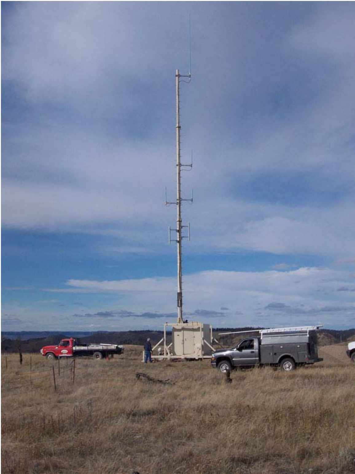
Example of a Shelter 8ft X 8ft X 8ft With Articulated Tower (approx. 60ft)
