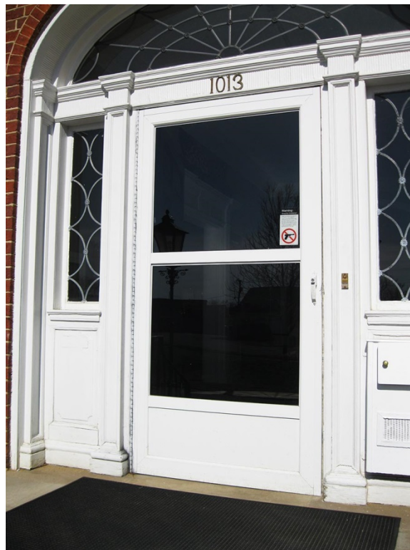
Current storm door on the front entrance of the Fredericksburg Battlefield Visitor Center – will be replaced with an white aluminum insulated door
