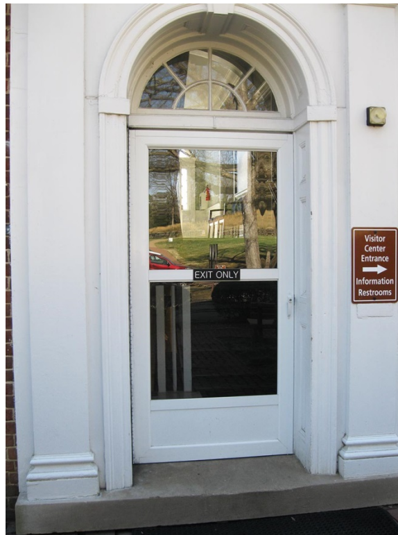
Current storm door on the rear entrance of the Fredericksburg Battlefield Visitor Center – will be replaced with an white aluminum insulated door
