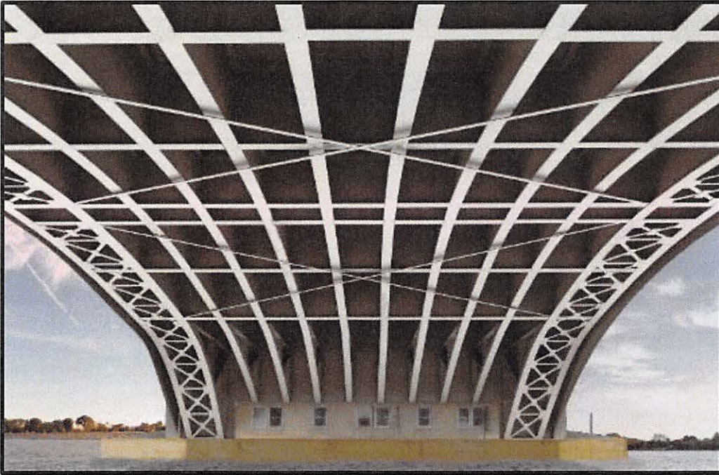
Conceptual rendering of variable depth steel girders (underside) under Alternative 1B
