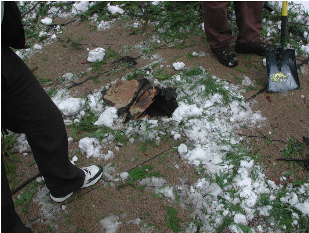
Photo 3 Hole in Roof , Building H-62
