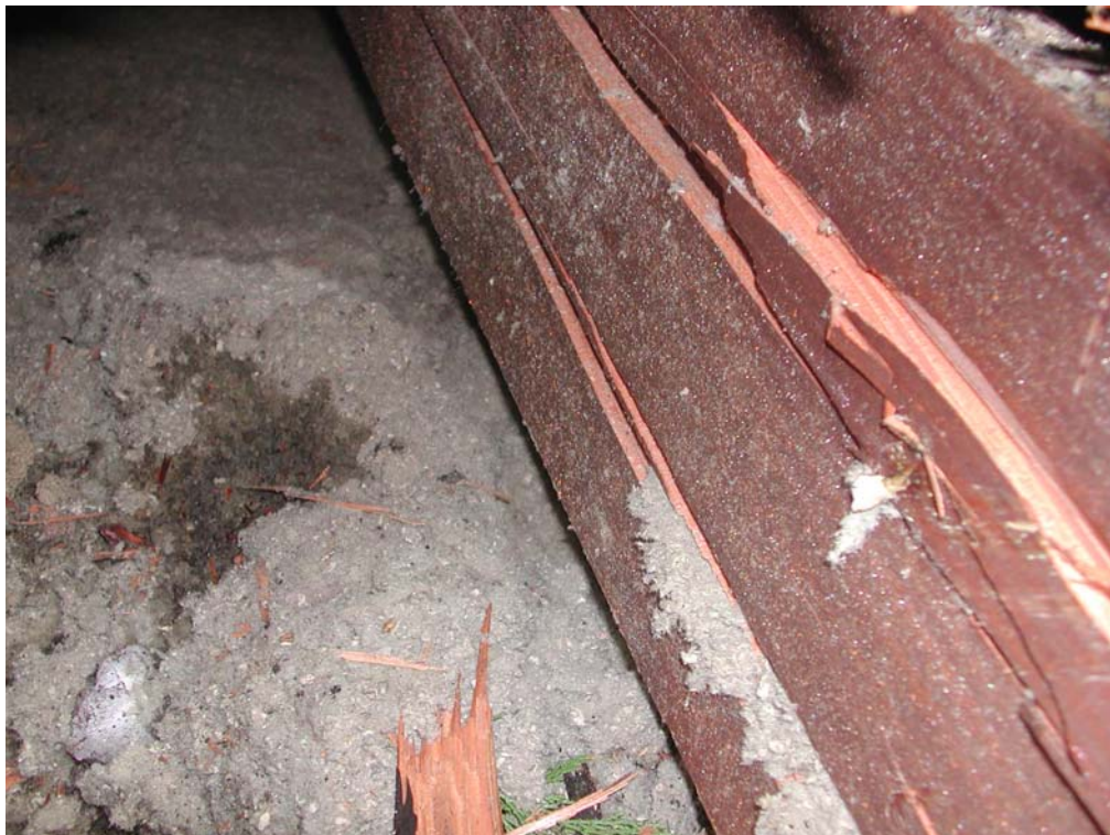
Photo 4 Cracked Roof Beam, Unit H-62
