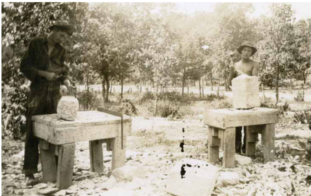
Figure 2-25. The CCC chiseled rocks to have smooth cleavage outside with clean edges for irregular courses, 1936. (OZAR Archives)
