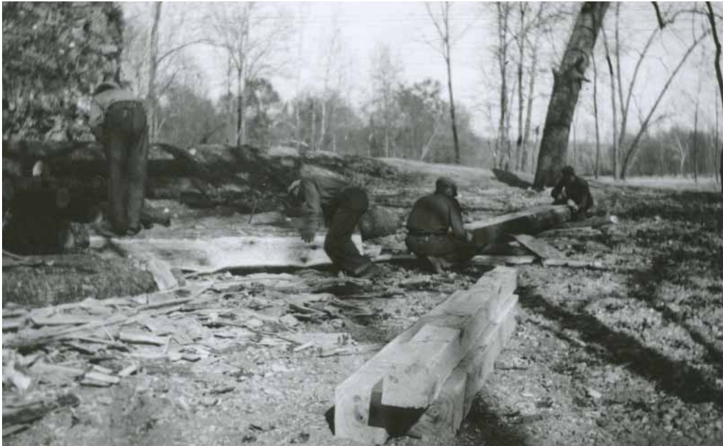
Figure 2-26. The CCC harvested trees on-site and cut dimensional timbers for buildings, date unknown. (OZAR Archives)
