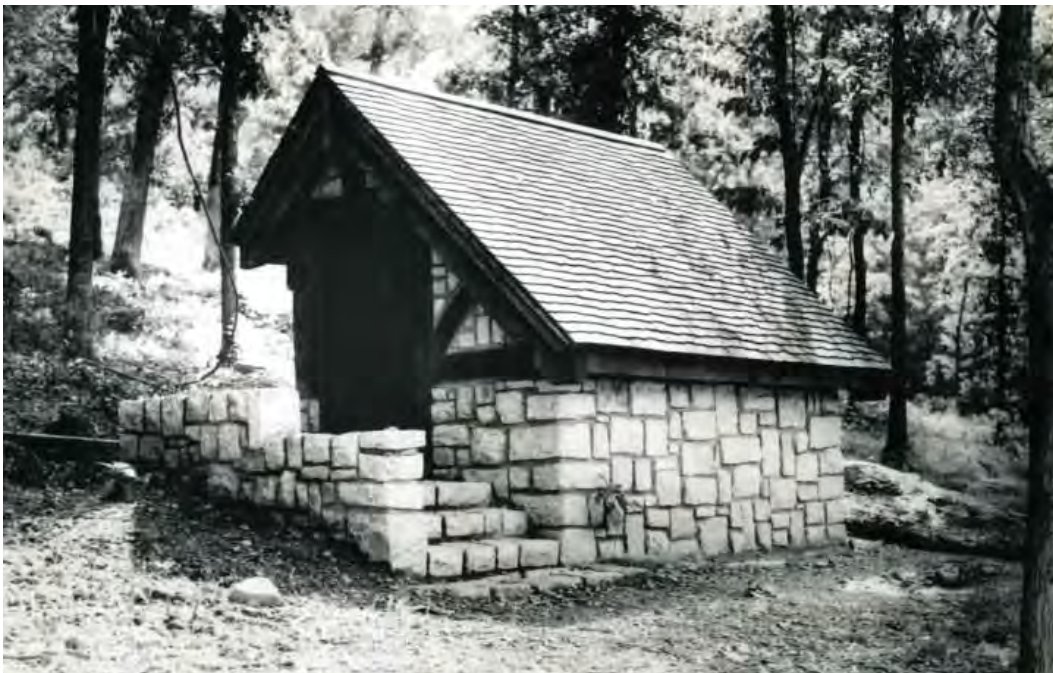
Figure 2-70. The CCC built a single story, open sided, Pump House (HS-443) with an asymmetrical gable roof and a combination of exposed timbers and irregular coursed cut stone walls, date unknown. (OZAR Archives)
