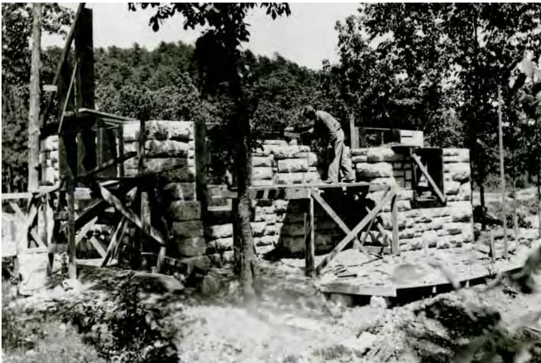
Figure 2-94. The cross gable Entrance Building (HS-432) had timber framing and irregular coursed cut stone wall, date unknown. (OZAR Archives)
