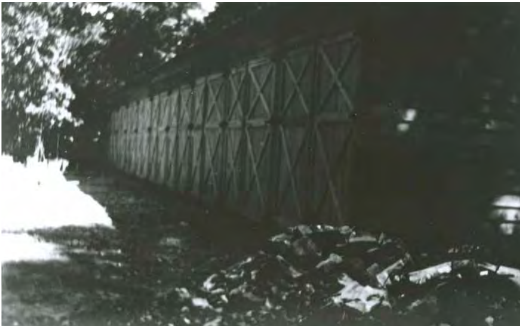
Figure 2-106. The CCC built a single story, wood framed Maintenance Garage (HS-419) with clapboard siding on a cut-stone foundation, date unknown. (OZAR Archives)
