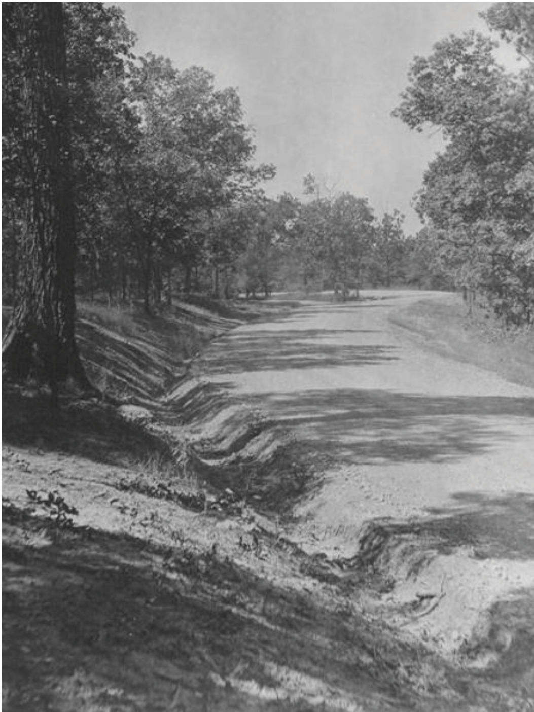
Figure 2-100. During construction of the Entrance Building (HS-432), the road was narrowed from 40' wide to 24' wide, date unknown. (OZAR Archives)
