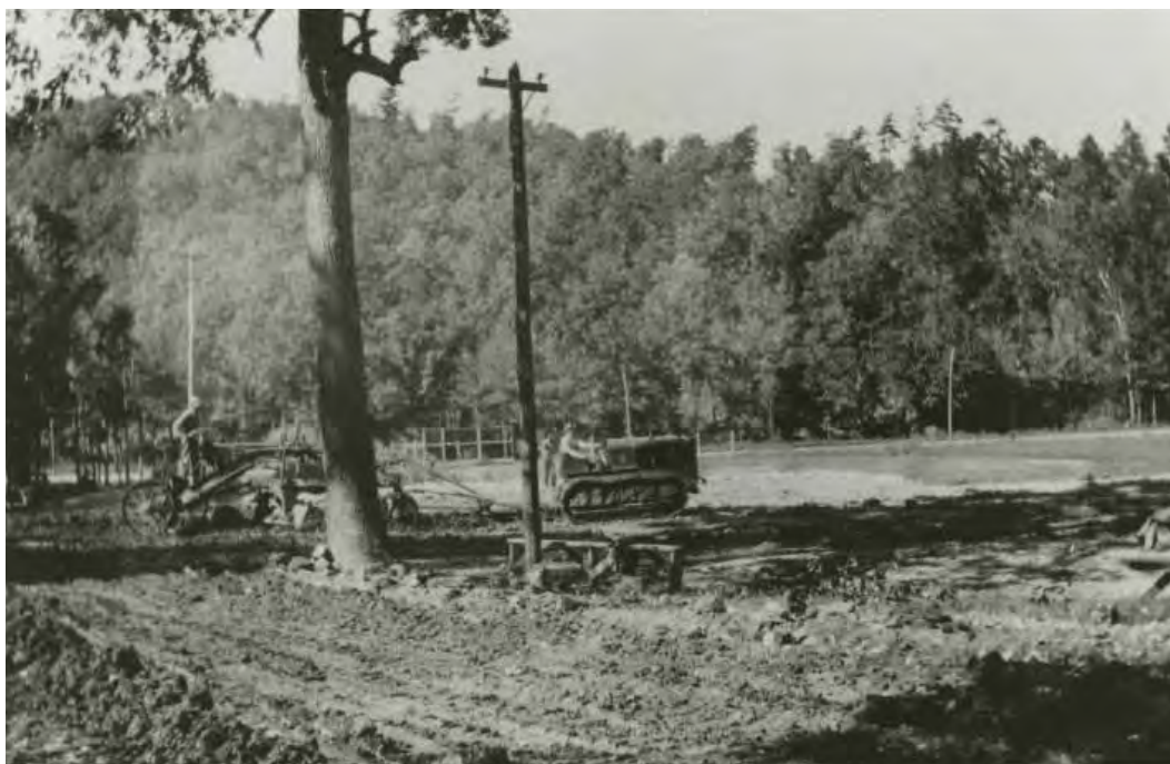
Figure 2-85. The CCC graded the Main Parking Area (HS-714), date unknown. (OZAR Archives)
