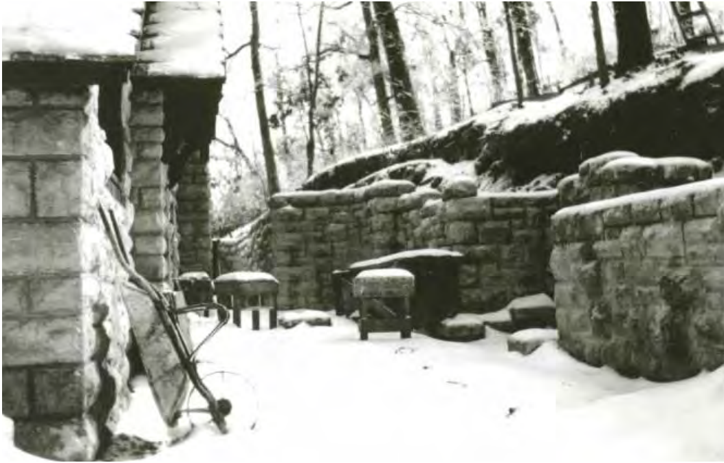
Figure 2-87. The CCC built the variable height Dining Lodge Retaining Wall and Fountain (HS-422A) with a circular, stepped fountain on axis with the rear door of the Dining Lodge (HS-422), date unknown. (OZAR Archives)
