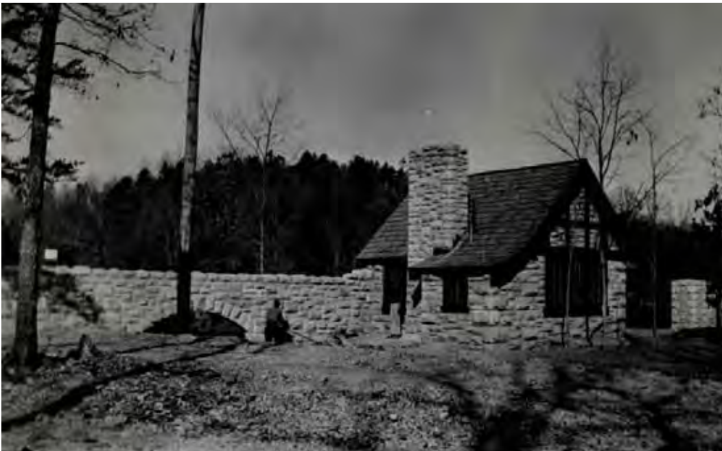
Figure 2-97. The Entrance Building (HS-432) was flanked with two forty foot walls with end piers and drainage arches, date unknown. (OZAR Archives)
