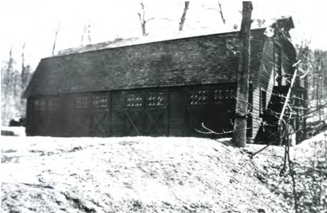
Figure 2-74. The Maintenance Shop (HS-417) was a two-story, three-room, gambrel roof building with a cut stone foundation and chimney, and exterior staircase, date unknown. (OZAR Archives)
