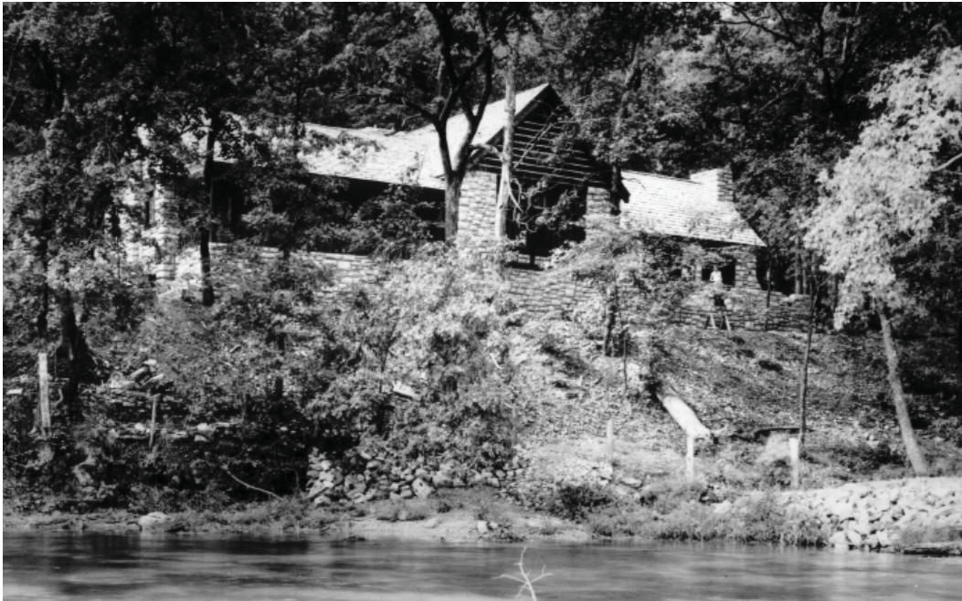
Figure 2-89. The cross gable Dining Lodge (HS-422) had timber framing with irregular coursed cut stone walls, two porches, a large flagstone entrance court, and a massive exterior stone chimney, date unknown. (OZAR Archives)
