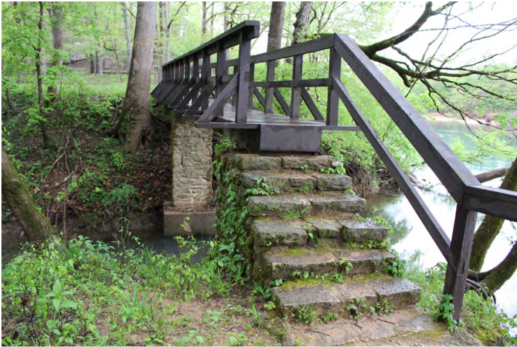
Figure 3-104. Chubb Hollow Foot Bridge (HS-456) wood decking and railing rebuilt, date unknown. Only the stone piers are contributing. (Mundus Bishop 2016)
