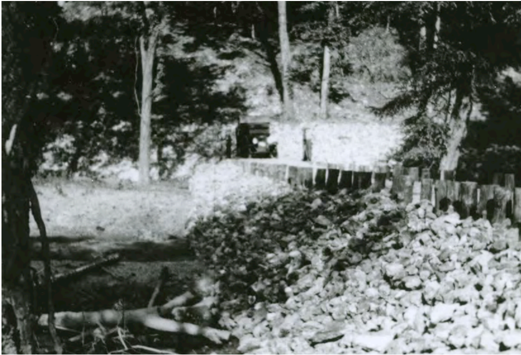
Figure 3-124. The Big Spring Stone Dikes (HS-711) were constructed of wood framing and rubble fill. They were also used as roads. Date unknown. (OZAR Archives)
