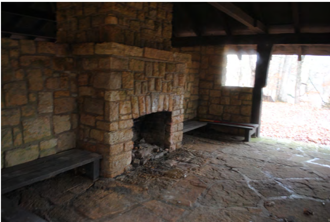
Figure 3-103. The Chubb Hollow Open Shelter House (HS-247) has a central chimney, and built-in plank benches. (Mundus Bishop 2015)
