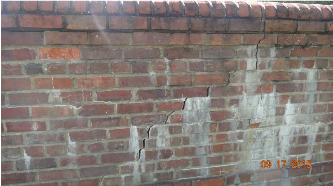
Image 1: Crack in wall north of iron gates.
