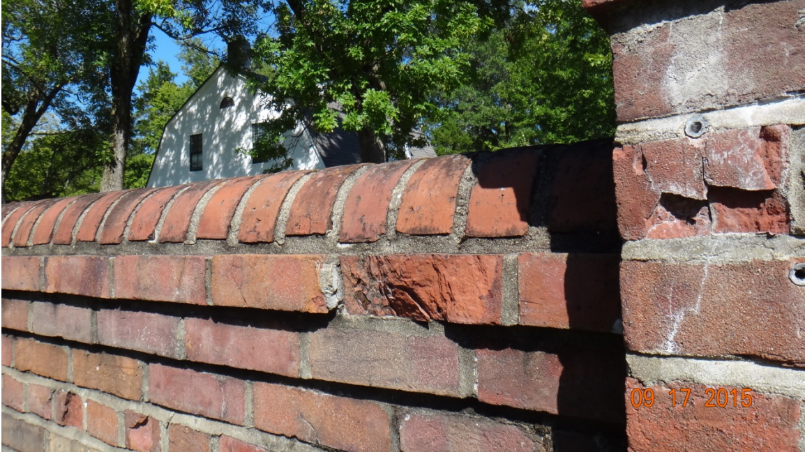
Image 2: Picture showing damaged brick. Indicative of numerous areas along the wall.
