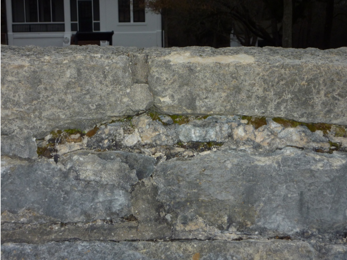
Image 3: Picture indicating areas of stone wall requiring repointing.
