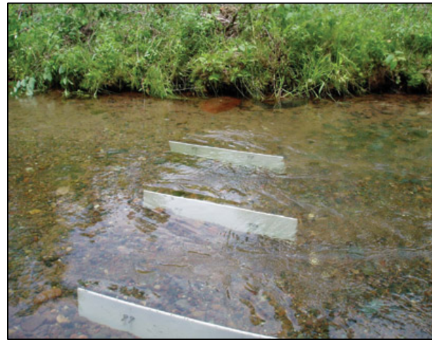
FIGURE 2-4. ENERGY REDUCTION VANES, NORTH FISH CREEK, WISCONSIN
