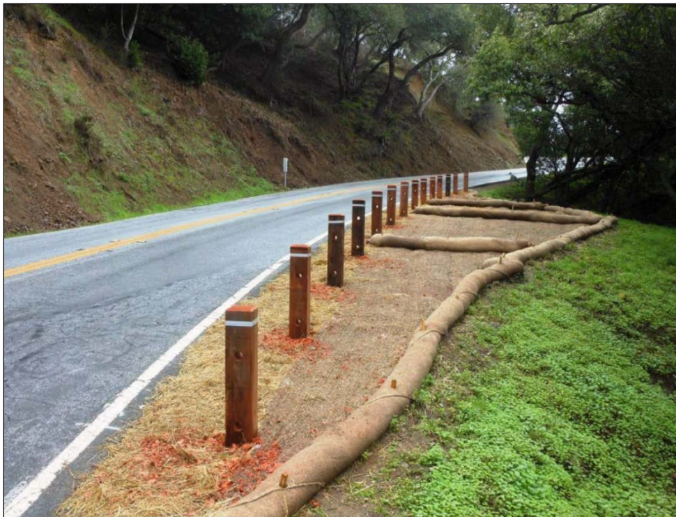
FIGURE 12. POST INSTALLATION AND EROSION CONTROL MEASURES
