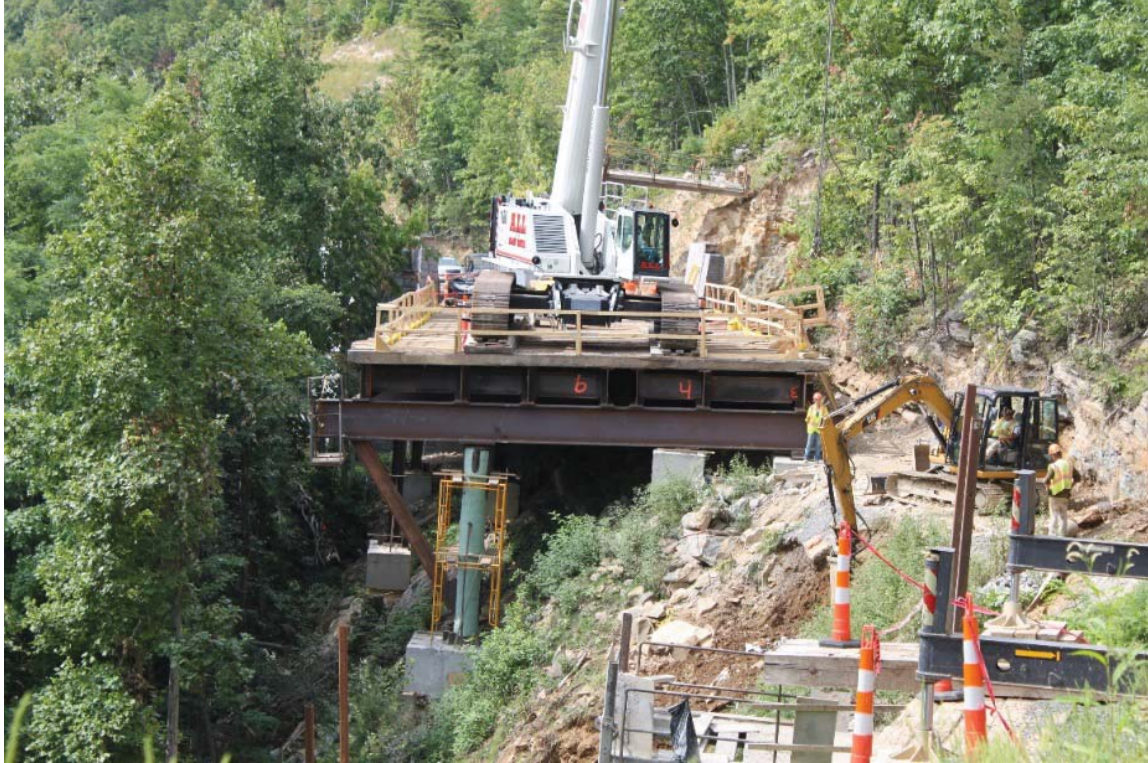
One of the bridges under construction on the Foothills Parkway.
