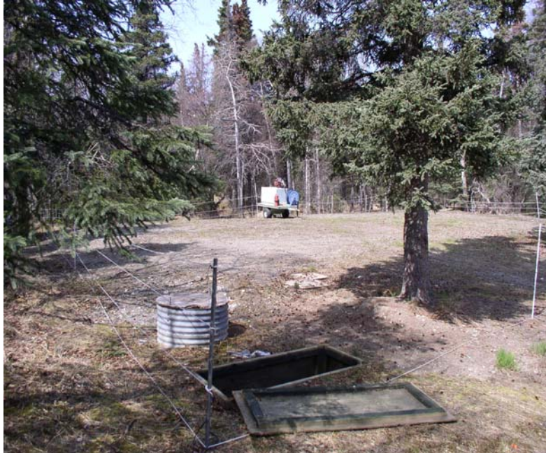
Photo 8. Brooks Camp leach field with open valve box
