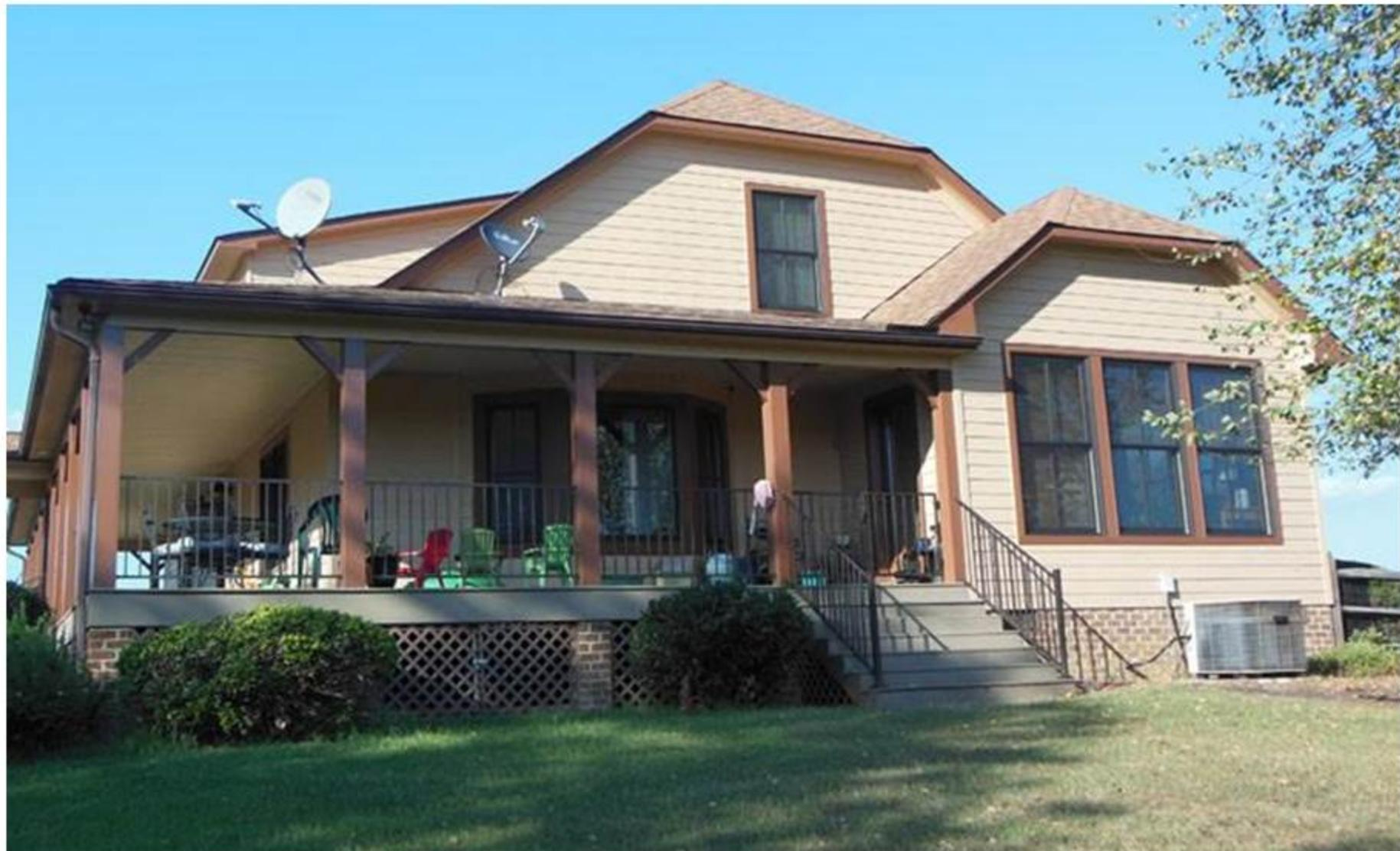
**South façade of existing (1996) dwelling, showing clipped-gables and pyramidal porch-roof—and onset of midafternoon shadows of adjacent trees—unsuitable for mounting solar array.**
