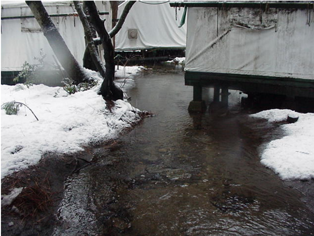
Photo 4 Flooding Inside Boy's Town Employee Residential Area
