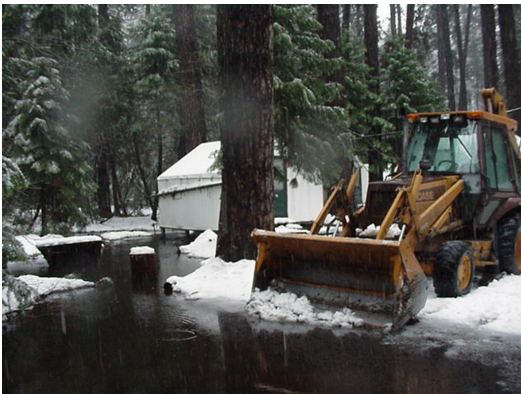
Photo 5 Flooding Inside Boy's Town Employee Residential Area
