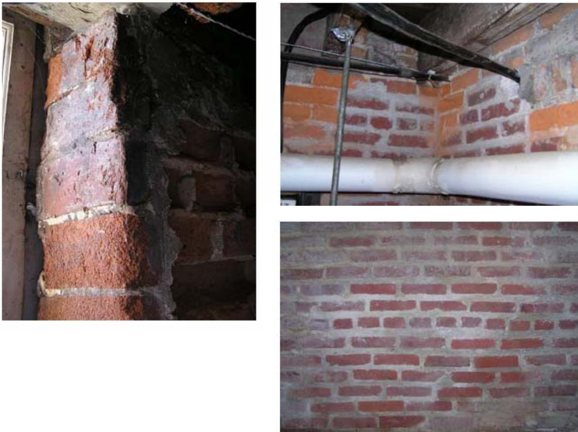
FIGURE 11: PHOTOGRAPHS OF ERODING HISTORIC BRICK AND OF MODERN BRICK SET IN WIDE PORTLAND CEMENT JOINTS IN FOUNDATION WALLS OF ARLINGTON HOUSE
