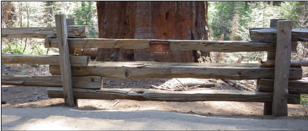
Example of fence in the Tuolumne Grove that was enhanced by addition of internal poles in 2015. The proposed new segment of fence will continue for 110 feet beyond the existing fence.
