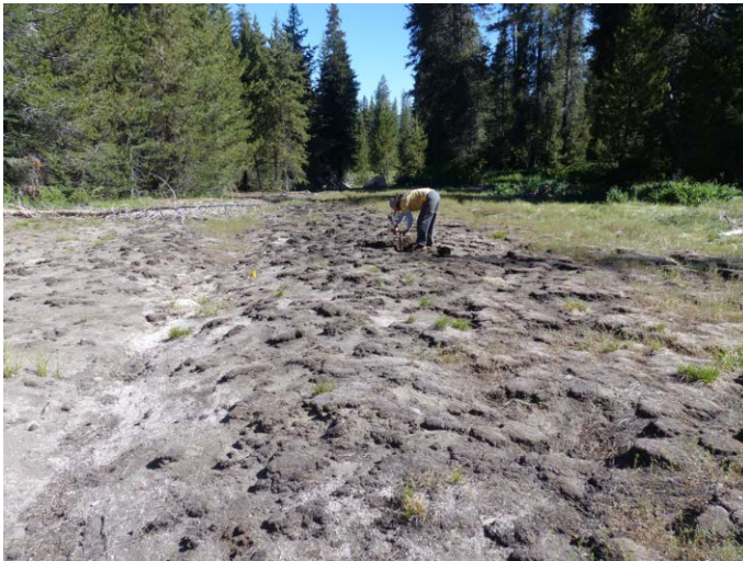
Photo 3. Dewatered Portion of Wetland
