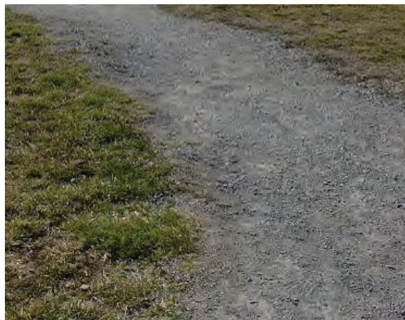
Figure 4- 5: Trail surface of crushed fines of limestone. (QEA)
