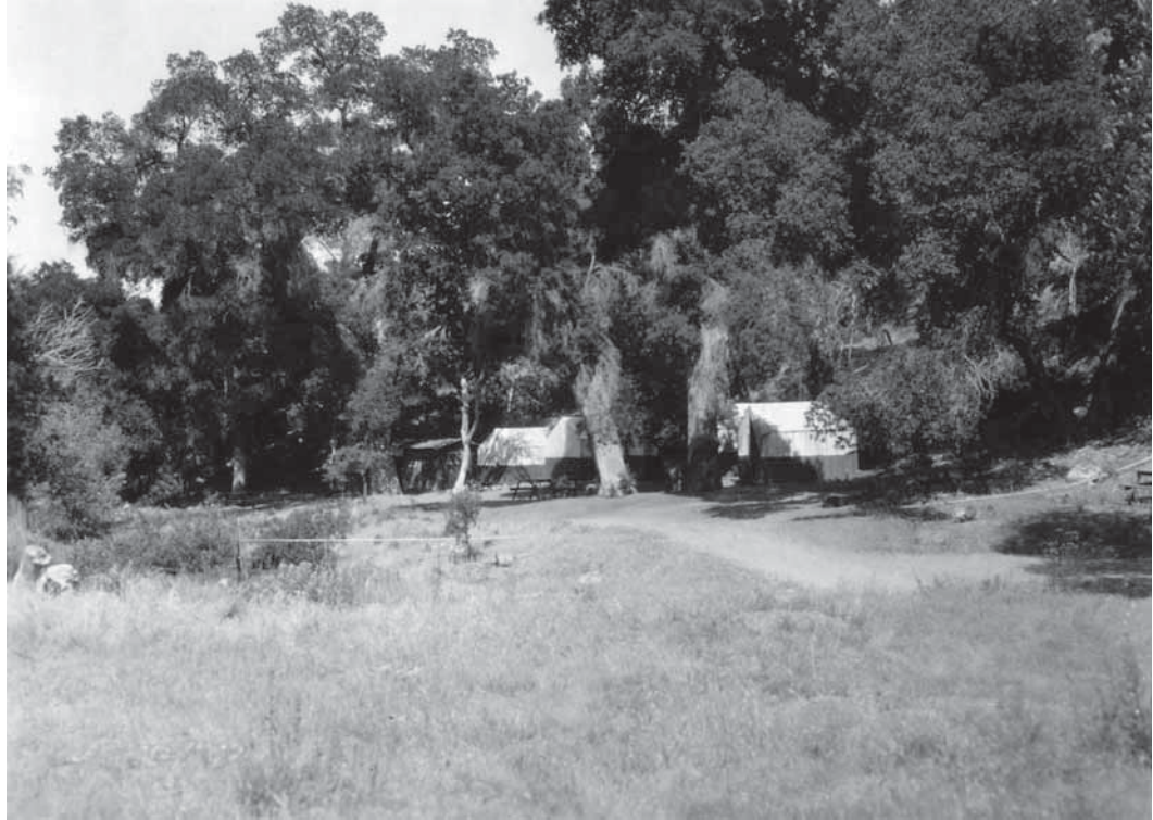
Figure 16. Lodge operators' cabins, looking east from lodge porch. Well is visible in shallow depression to left. These cabins are in approximate location of the present headquarters buildings. [Included in report of Dunn to Hommon, August 10, 1929, PINN Coll., RG 79, Entry 7, Box 607, NARA II.]
