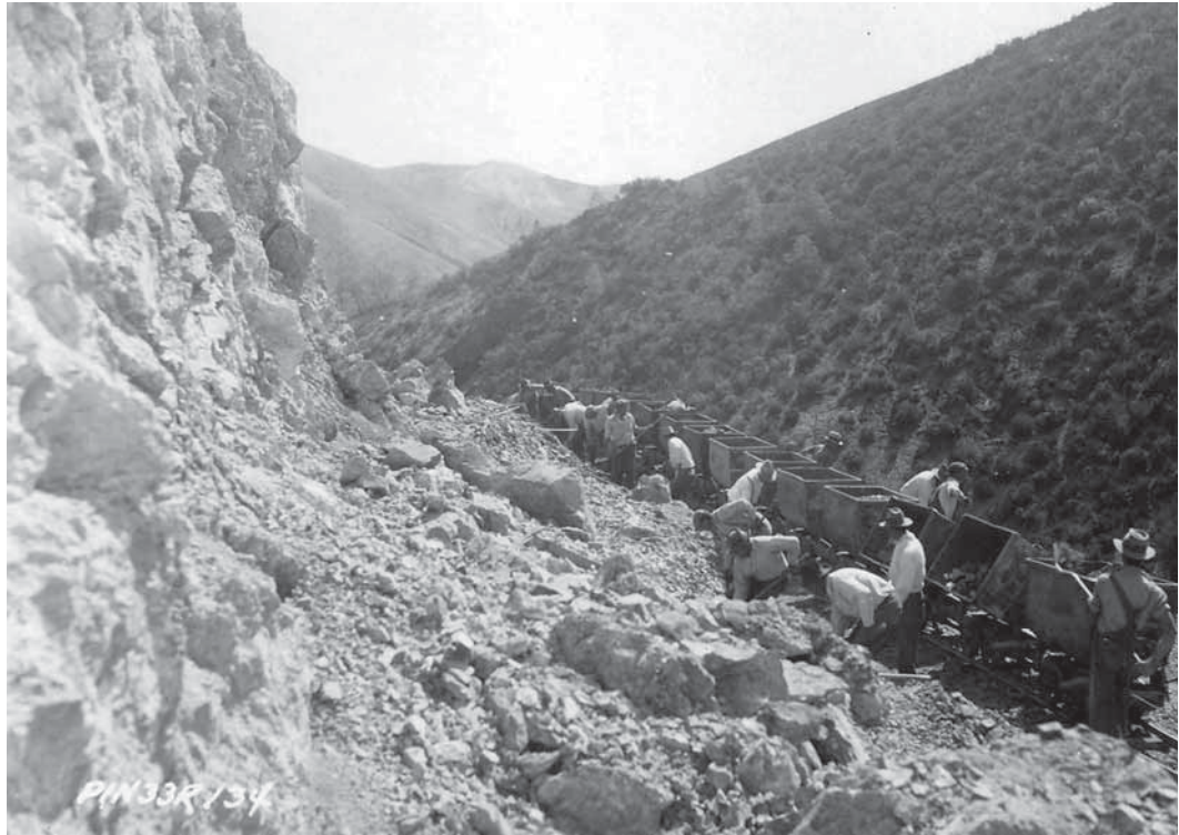
Figure 26. Local laborers working on the new Bear Gulch entrance road in 1932. Ore cars were borrowed from the nearby New Idria mercury mines to convey waste rock off the cut slope. [Mus. Coll. PINN 4372, PNM.]
