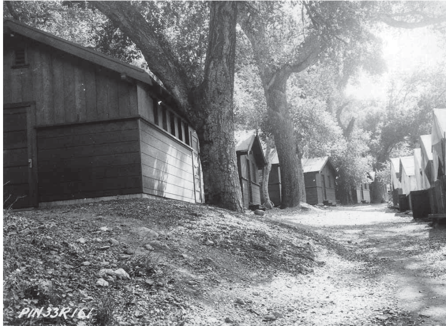
Figure 24. Laborers village in Bear Gulch, 1933. Many of the hardwalled buildings to left are still extant and being used for administrative purposes by Park staff. Most of these were faced up to the windowsills with stone by the Civilian Conservation Corps a few years later. The tent cabins to the right were removed shortly after the road project was completed. [Included in E.A. Kittredge, "Final Report on Construction of Entrance Road," April 15, 1933, Mus. Coll. PINN 3658, PNM.]
