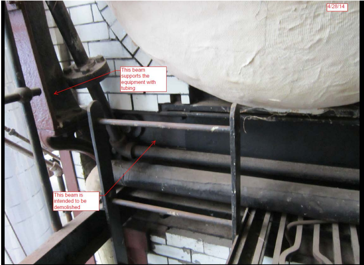
FIGURE 4 - Tubing above boiler support
