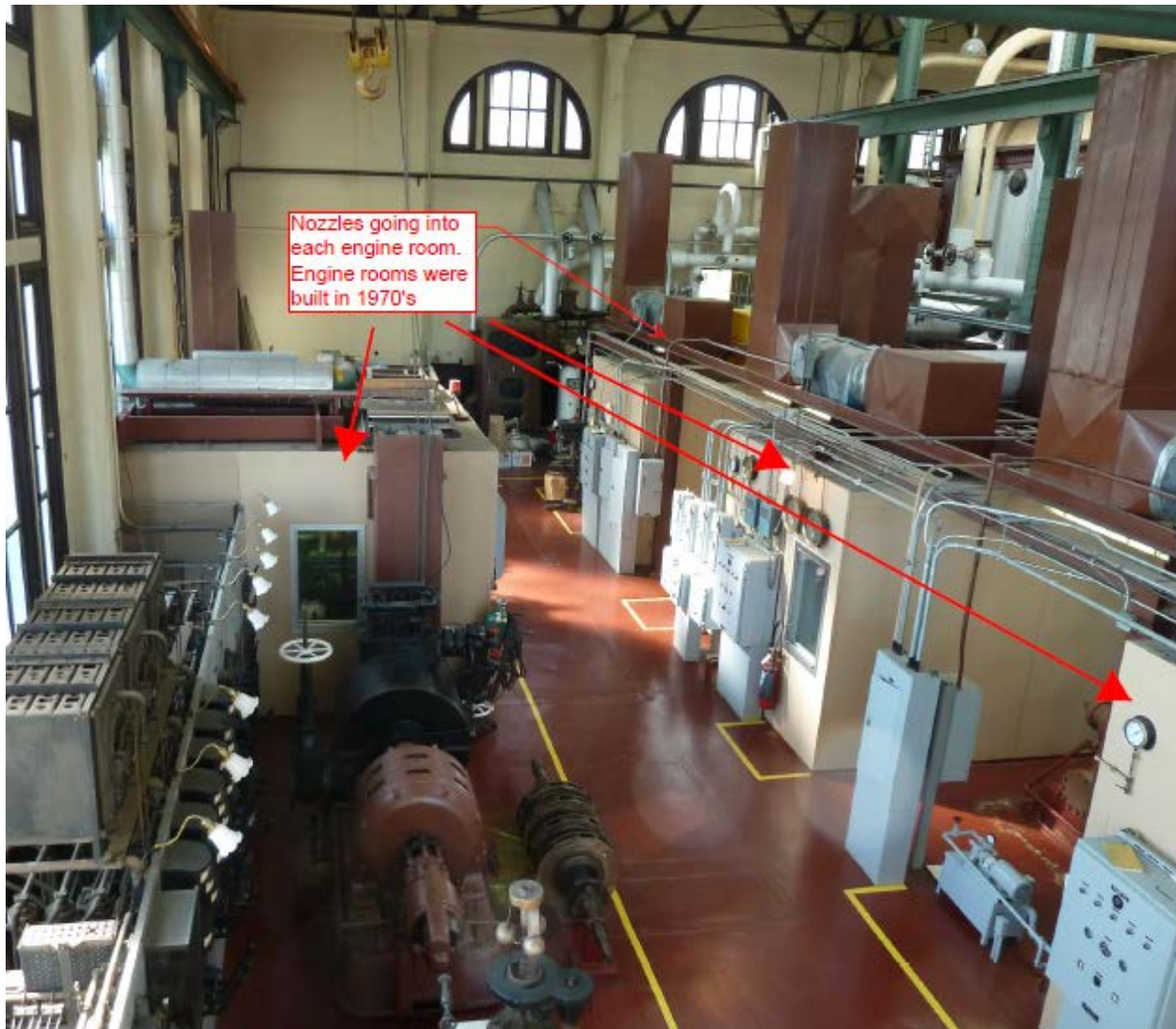
FIGURE 23 - Existing conduits and utility frame.
