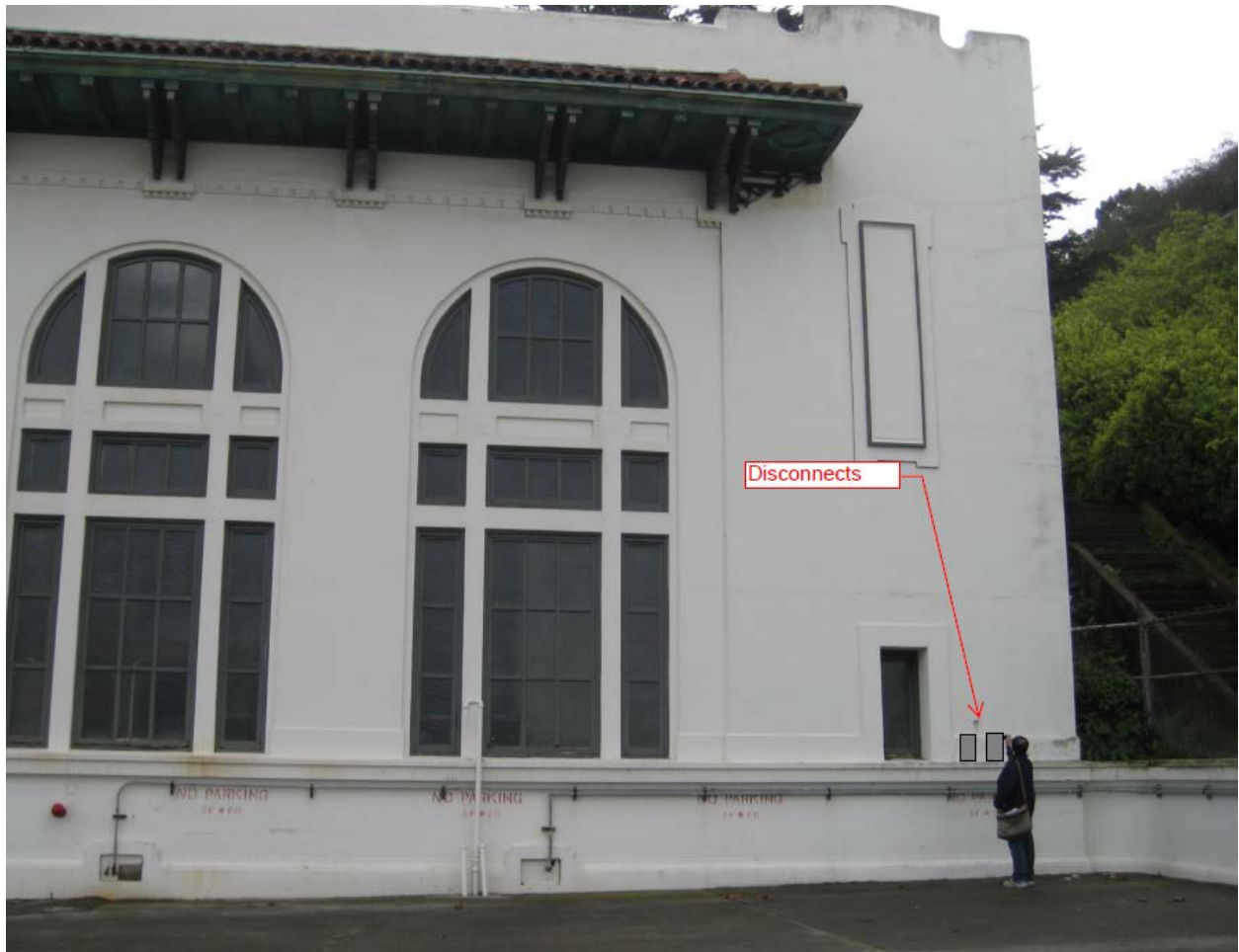
FIGURE 25 – Location of the new disconnect switches on northern façade of building.
