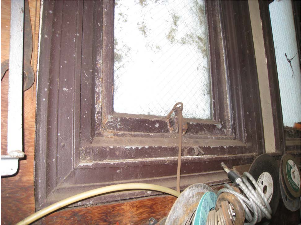
FIGURE 20 – Existing window interior trim
