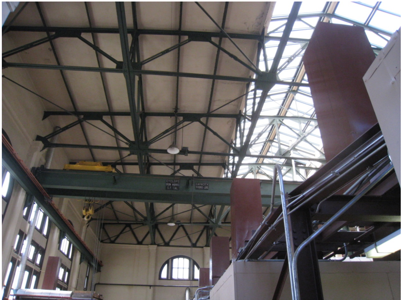
FIGURE 12 - Roof deck as seen from the interior.
