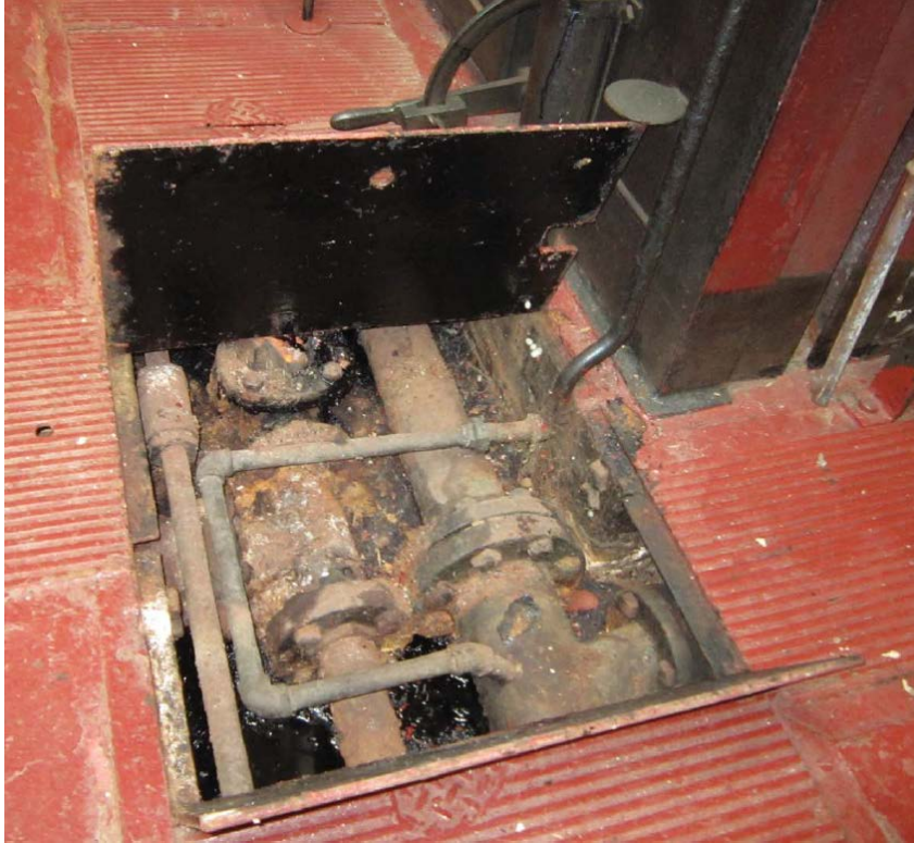
FIGURE 7 - Boiler trench with trench plates removed
