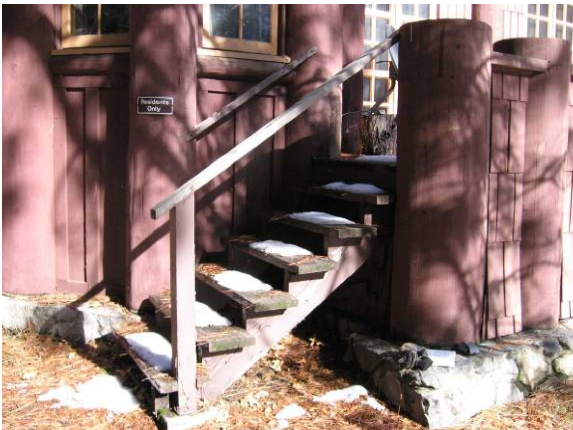
South deck stairs in need of replacement.
