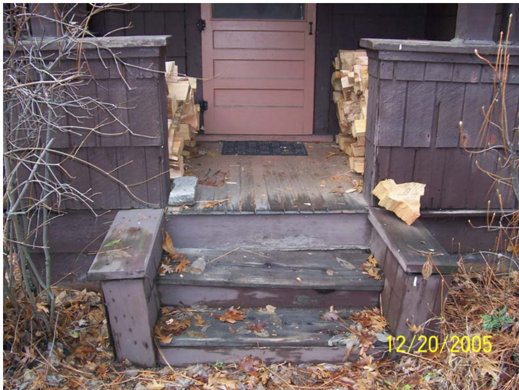
Photo 2 Residence #6 Front Steps
