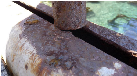
Photo 32. View of Scorpion Pier fractured weld connection at guardrail post base.
