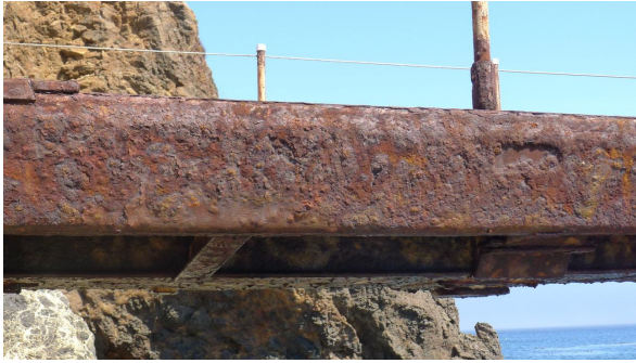
Photo 31. View of Scorpion Pier corroded exterior stringer at shore abutment.
