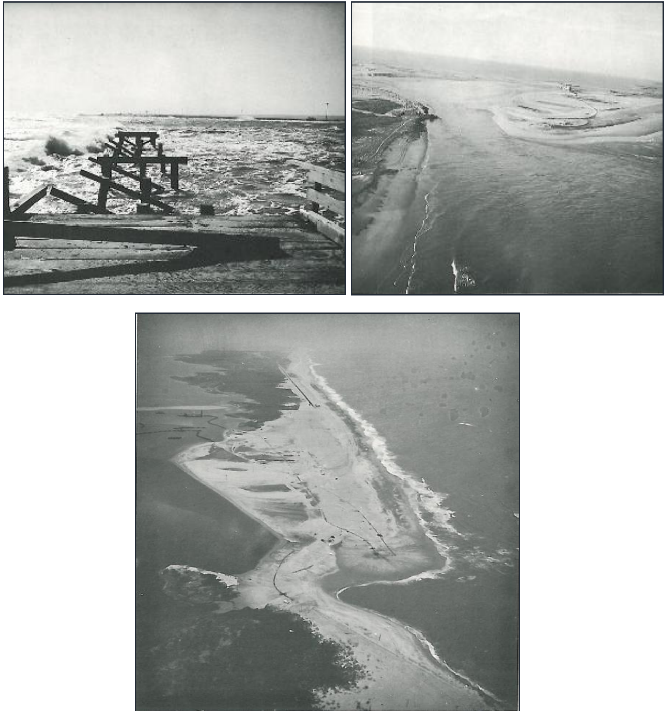
Figure 1.7. In March 1962, the mid-Atlantic northeaster of record, Ash Wednesday storm, breached the dunes at Buxton and opened an inlet within the Proposed Action Area. A temporary timber bridge was built over the inlet to restore access. However, a northeaster during the period 25 November to 3 December 1962 destroyed the bridge. The images show the inlet at Buxton (upper left) looking south (5 December 1962). Local interests (non-federal) closed the breach between (upper right) 29 January 1963 and (lower) 21 February 1963. The borrow source was in Pamlico Sound in close proximity to the project site. (From USACE 1963, Appendices 6-19)
