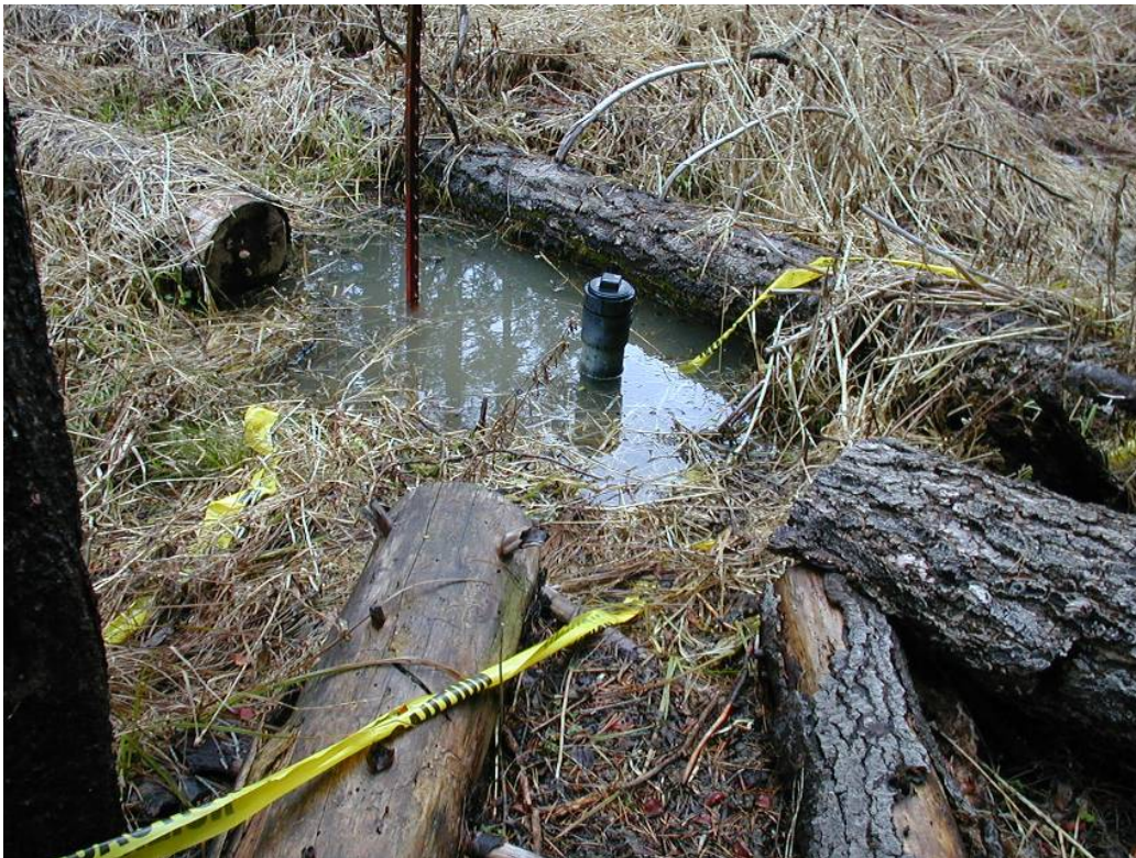
Photo 2 Site of the Leak
