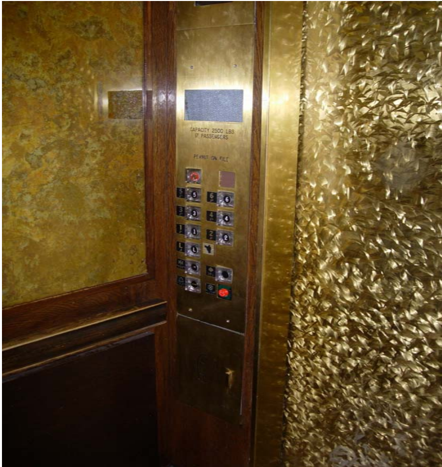
Ahwahnee Elevator Cab Control Panel
