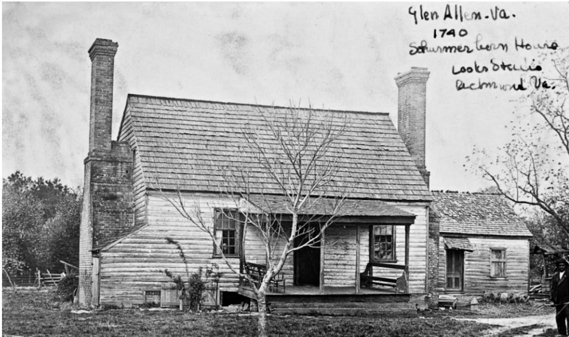
Figure 14. Schurmerberg House. Glen Allen, Virginia. (Destroyed). Deep chimneys, with weatherings on three faces. Valentine Museum. (Date unknown).
