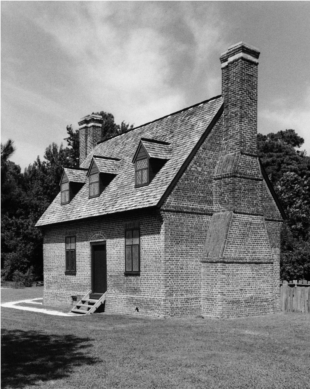
Figure 15. Lynnhaven (Wishart) House. Virginia Beach, Virginia. Large chimney, with foundation stepped at grade. National Register of Historic Places. (1969).
