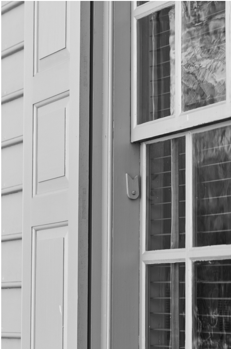
Figure 29. Charlton's Coffeehouse. Williamsburg, Virginia. Pivoting cleat to hold lower sash open. Jennifer Glass. (2012).
