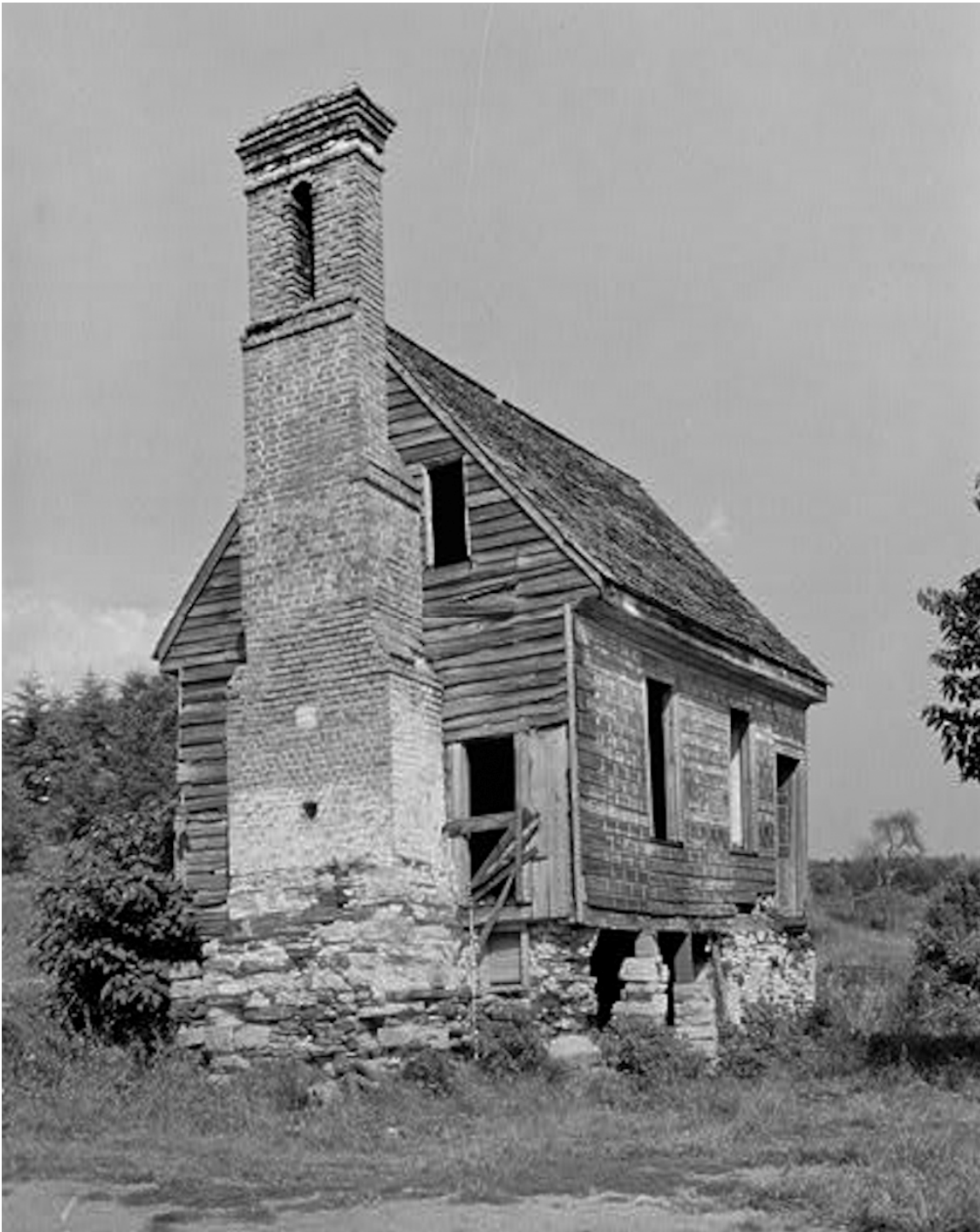
Figure 12. Merchant House. Dumfries, Virginia. (Destroyed). Stone foundation of chimney extends above finished floor. HABS, Library of Congress. (1933).
