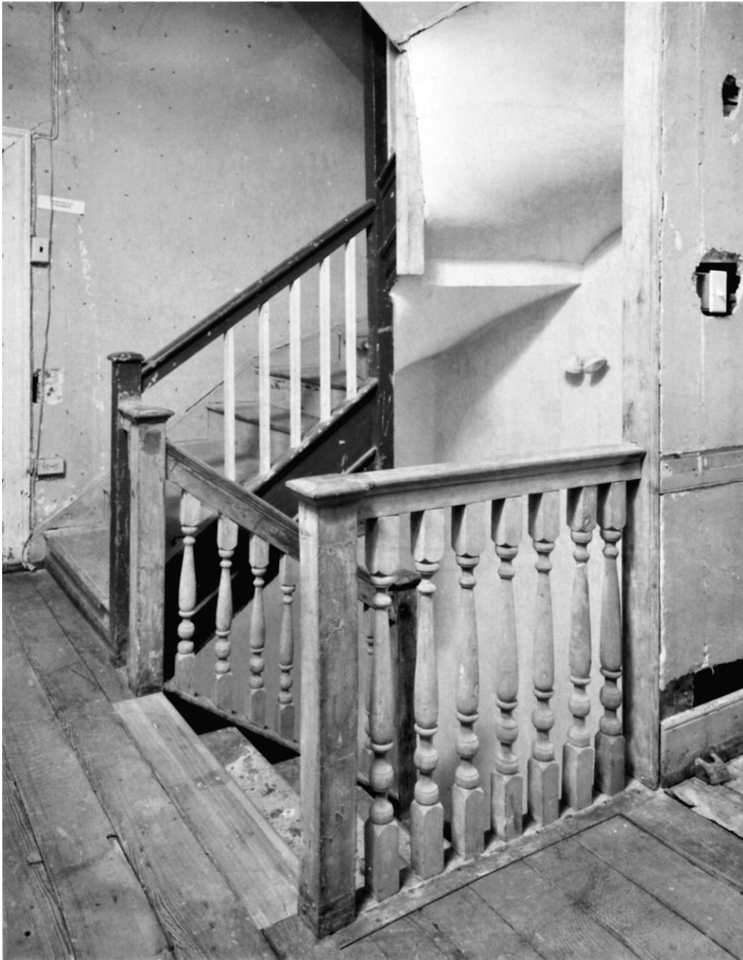
Figure 36. Charles Carroll House. Annapolis, Maryland. Closed-string stair, with cap details for raking and horizontal railings. Willie Graham. (1997).
