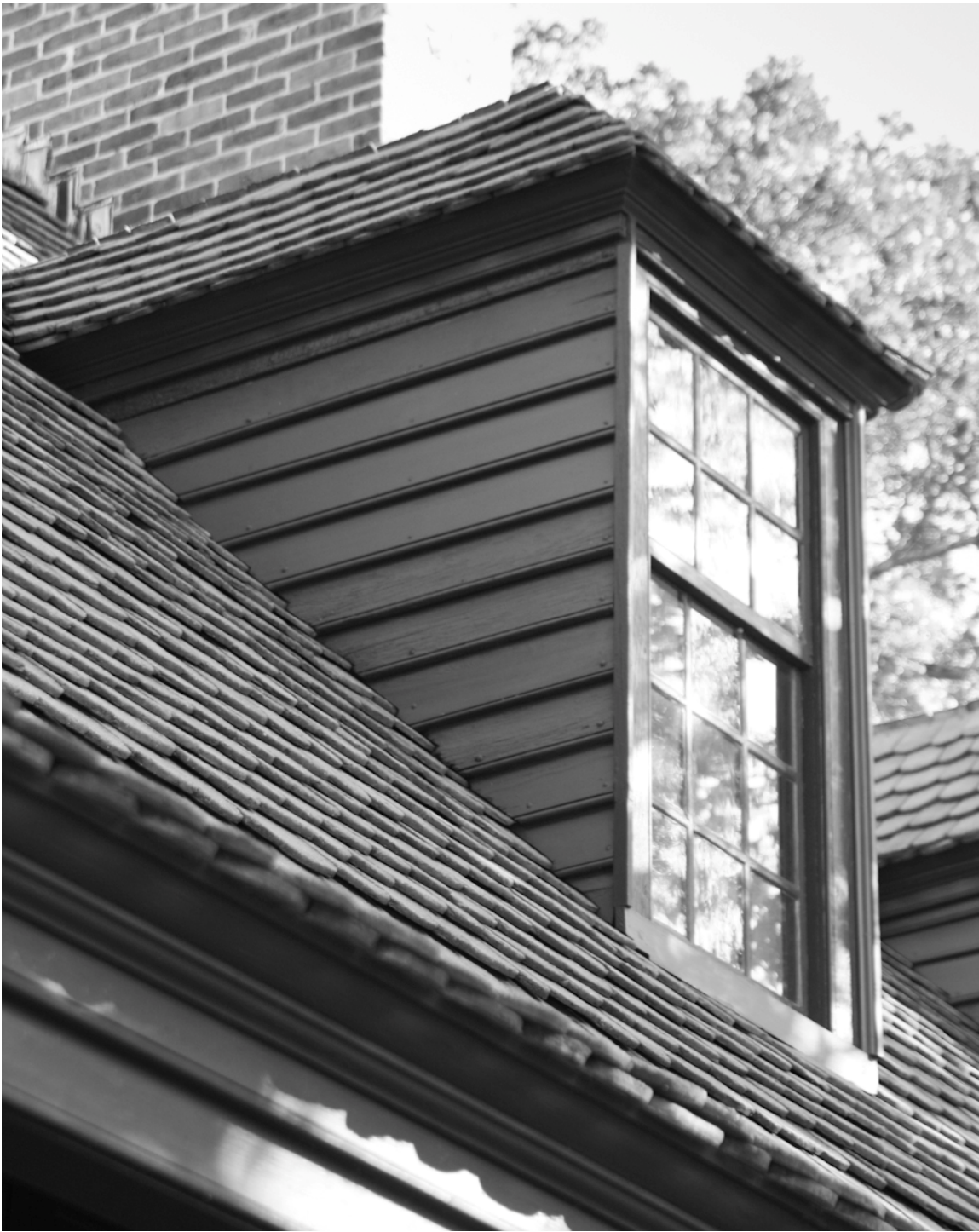
Figure 31. Wetherburn's Tavern. Williamsburg, Virginia. Beaded weatherboards on dormer cheeks. Jennifer Glass. (2012).
