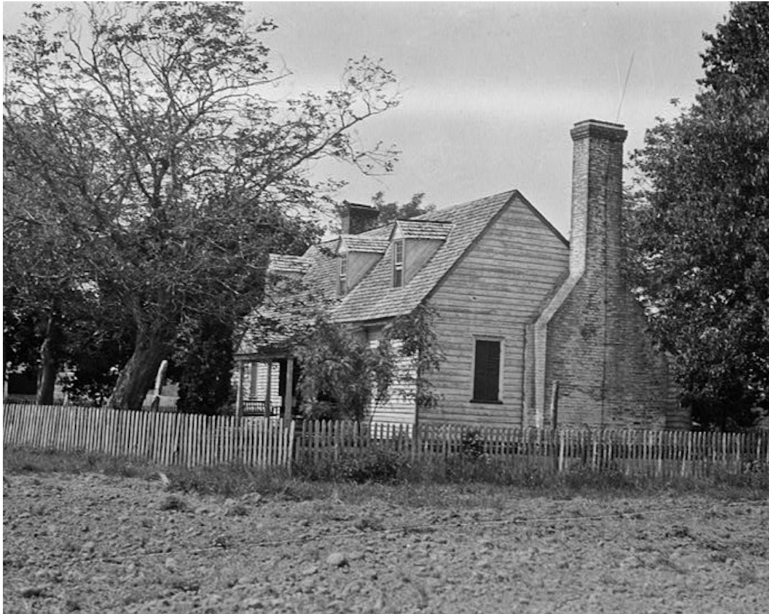
Figure 21. Linden Farm. Richmond County, Virginia. Side elevation shows shed rafters attaching at ridge of main roof. National Register of Historic Places. (1976).
