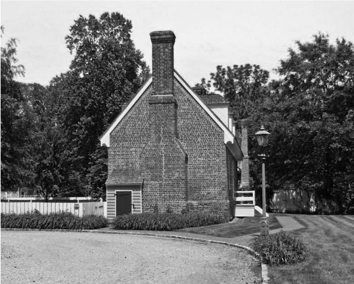
Figure 16. Eagle's Nest (Claybank). Charles City County, Virginia. Weatherings below stack on three sides. DHR .
