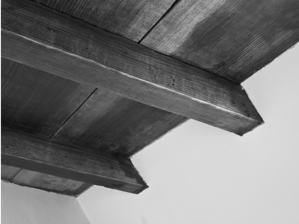
Figure 39. Lynnhaven House – Virginia Beach, Virginia. Exposed collar ties, eased edges. Jennifer Glass. (2012).
