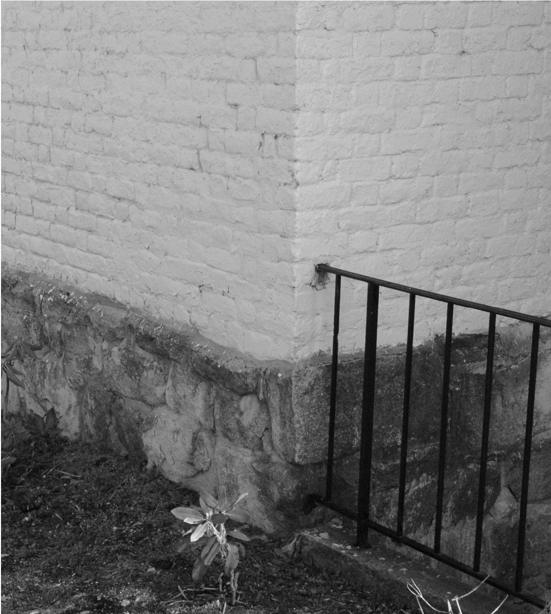
Figure 13. “The Chimneys.” Fredericksburg, Virginia. Brick chimney borne on a stone foundation. Jennifer Glass (2012).
