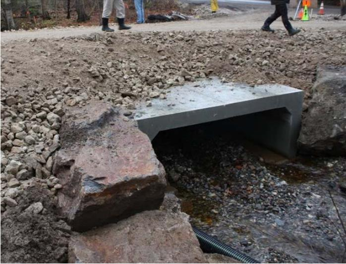
Figure 4. Typical six feet wide x five feet tall precast box culvert, stone wing walls, no guardrail
