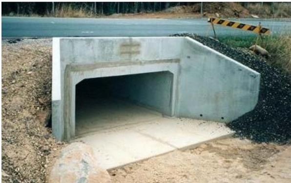
Figure 3. Typical six feet wide x five feet tall precast box culvert, cement wing walls, no guardrail
