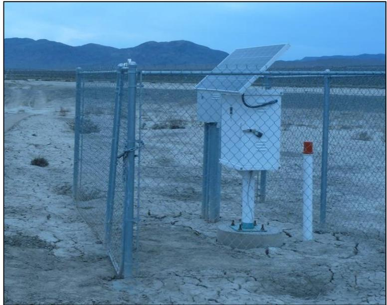
**Photograph 1.** Existing solar impressed current system with chain link fence perimeter.
