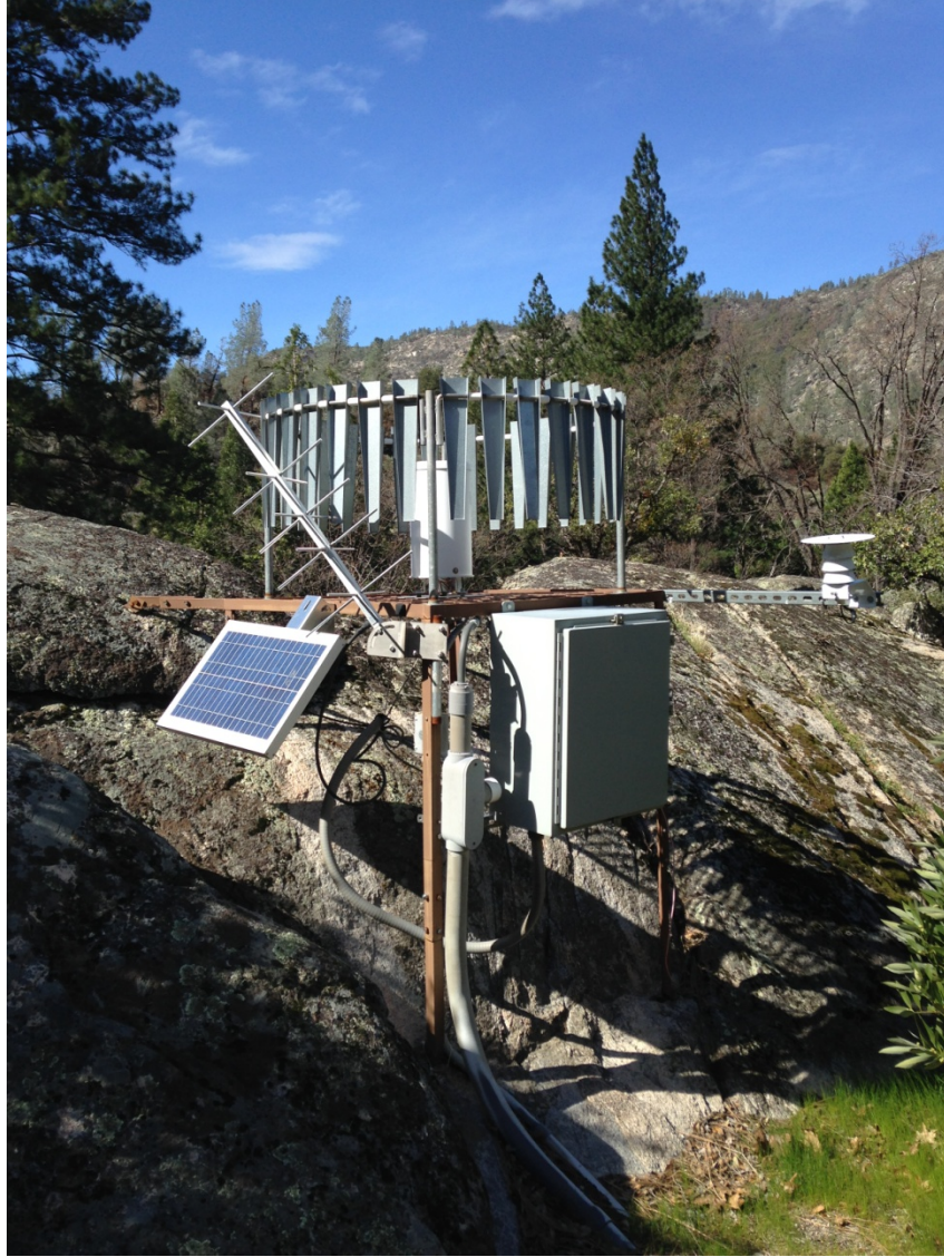
Figure 4: Existing weather station overlooking Evergreen Road (to be removed). Solar panel, radio and box will be repurposed for new station. A new precipitation gage will be purchased.
