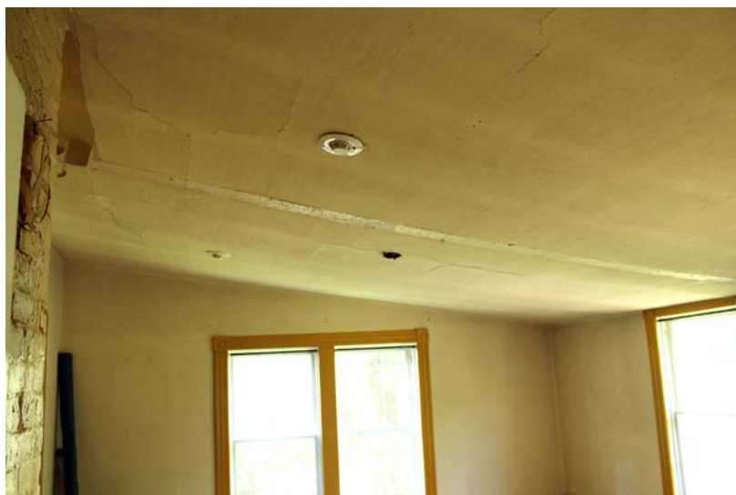
Existing condition of plaster ceiling below metal roof (Room 211, Dr. Hubbell's Bedroom)
