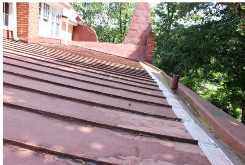
Lack of expansion joints on low-sloped roof results in frequent failures (Southeast Side)
