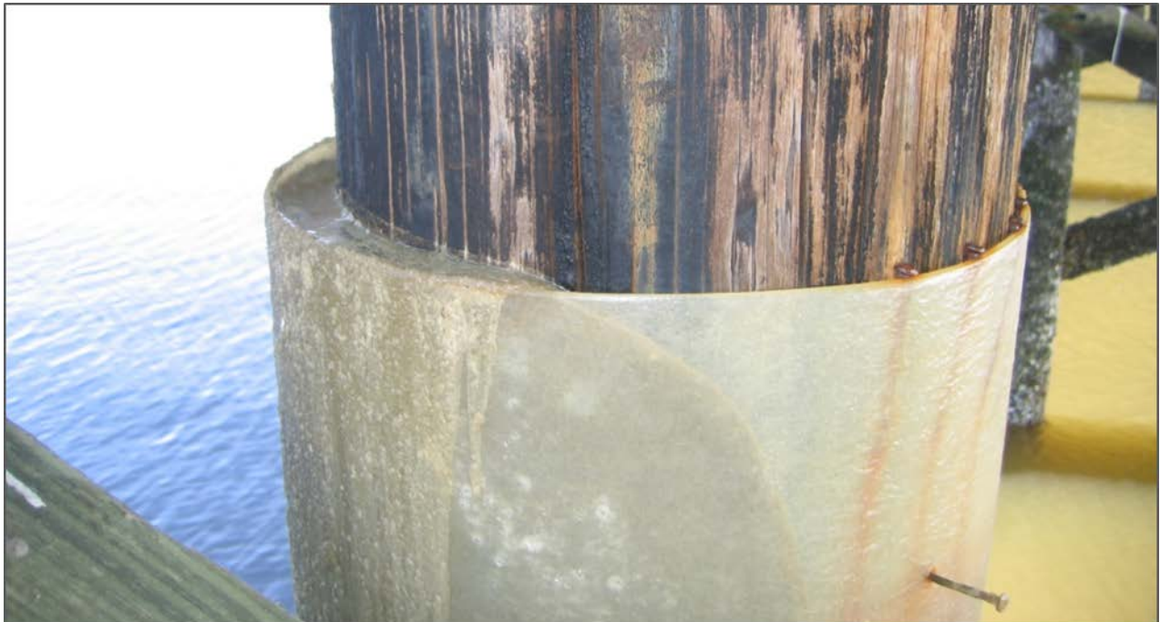
Figure 3. An existing FRP jacket is shown.
