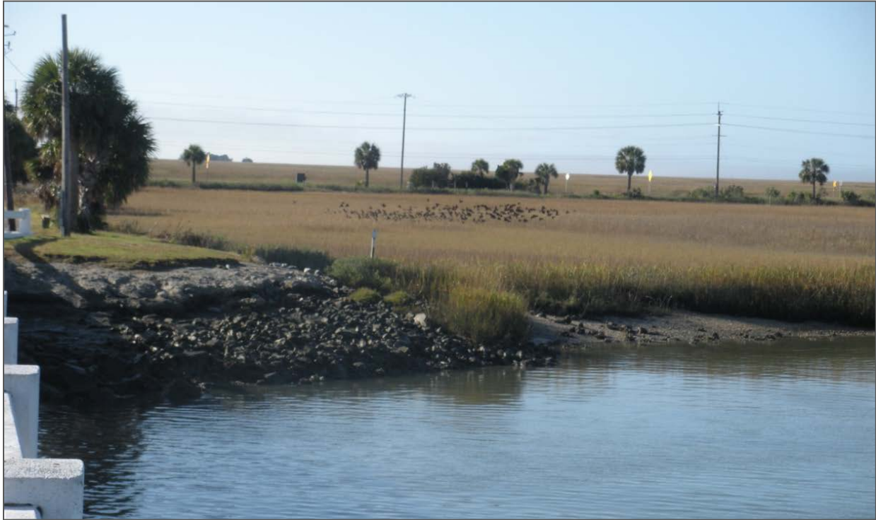
Figure 10. The tidal marsh is shown adjacent to the riprap protecting the bridge abutment.
