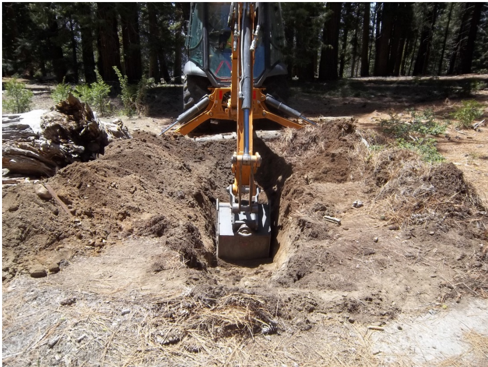
Photo 6: Trench T1 being dug
